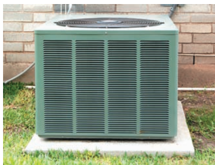
This air conditioner transfers heat energy from the cool indoors to the hot exterior.
