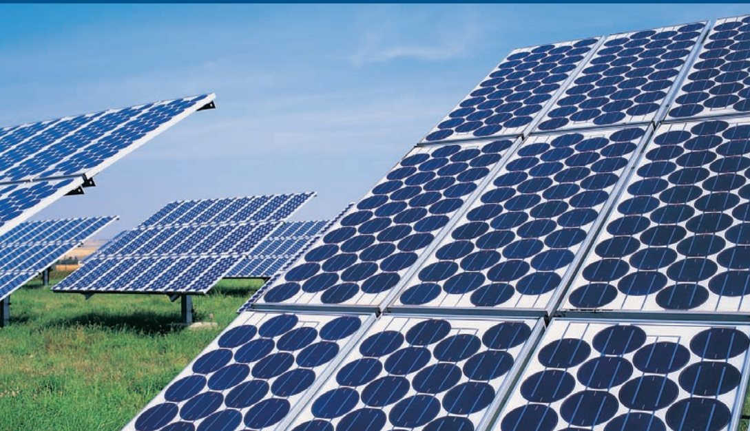
These solar cells are photovoltaic cells, meaning that light creates a voltage—a potential difference.
