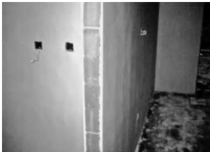
Figure 10.7. Partition wall, wet finish with gypsum plaster.
