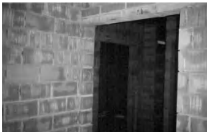
Figure 10.1. Heavy-weight partition wall, masonry.
