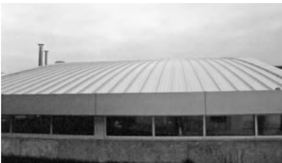
Figure 7.6. Self-bearing aluminium cover.
