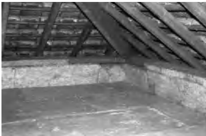
Figure 6.35. Insulation at ceiling level.
