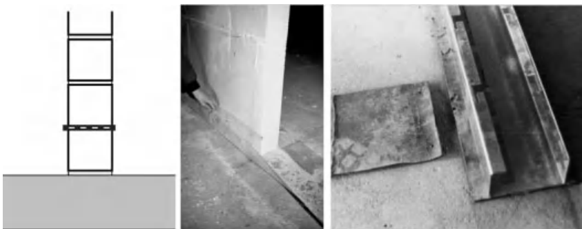
Figure 10.3. Partitions walls, combating cleaning water suction: on the left for masonry walls, in the middle for gypsum block walls, on the right for lightweight walls.
