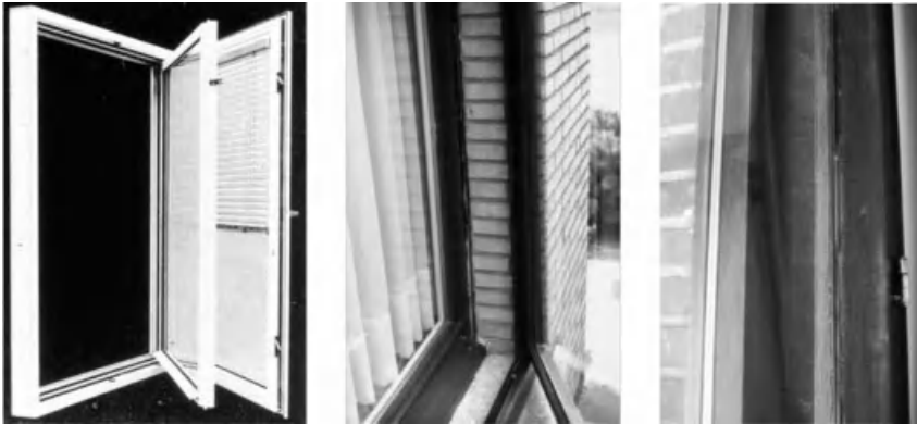
Figure 8.28. Left: Twofold window. Middle and right: double windows.
