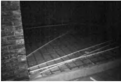
Figure 10.9. Floor slab with plastic draw-in pipes on it.
