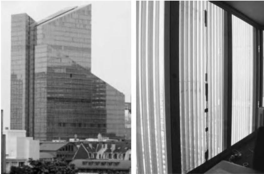
Figure 8.36. On the left the office building, on the right a bay of the double skin façade with the solar shading closed.
