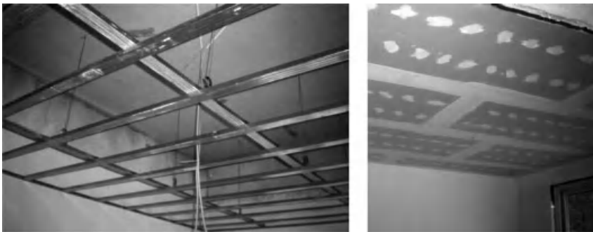
Figure 10.15. Closed gypsum board hung ceiling.
