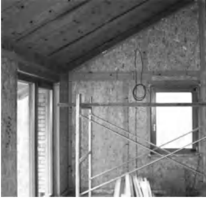
Figure 1.4. Taped OSB as air barrier.
