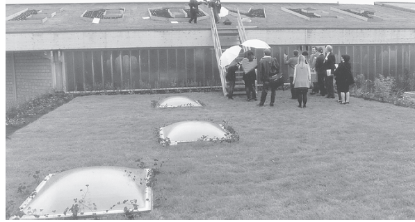
Figure 3.20 The ecoroof atop Ecover's headquarters helps meet the company's goal of a green factory producing green products. (Project: Ecover. Photo: Peter Malaise.)
