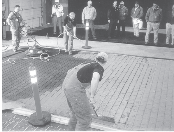
Figure 5.20 Decorative color coatings for asphalt can lighten the surface, decreasing heat-island effects. Integral color, mixed into hot asphalt, is also becoming available. (Photo: StreetPrint, Scott Hind.)
