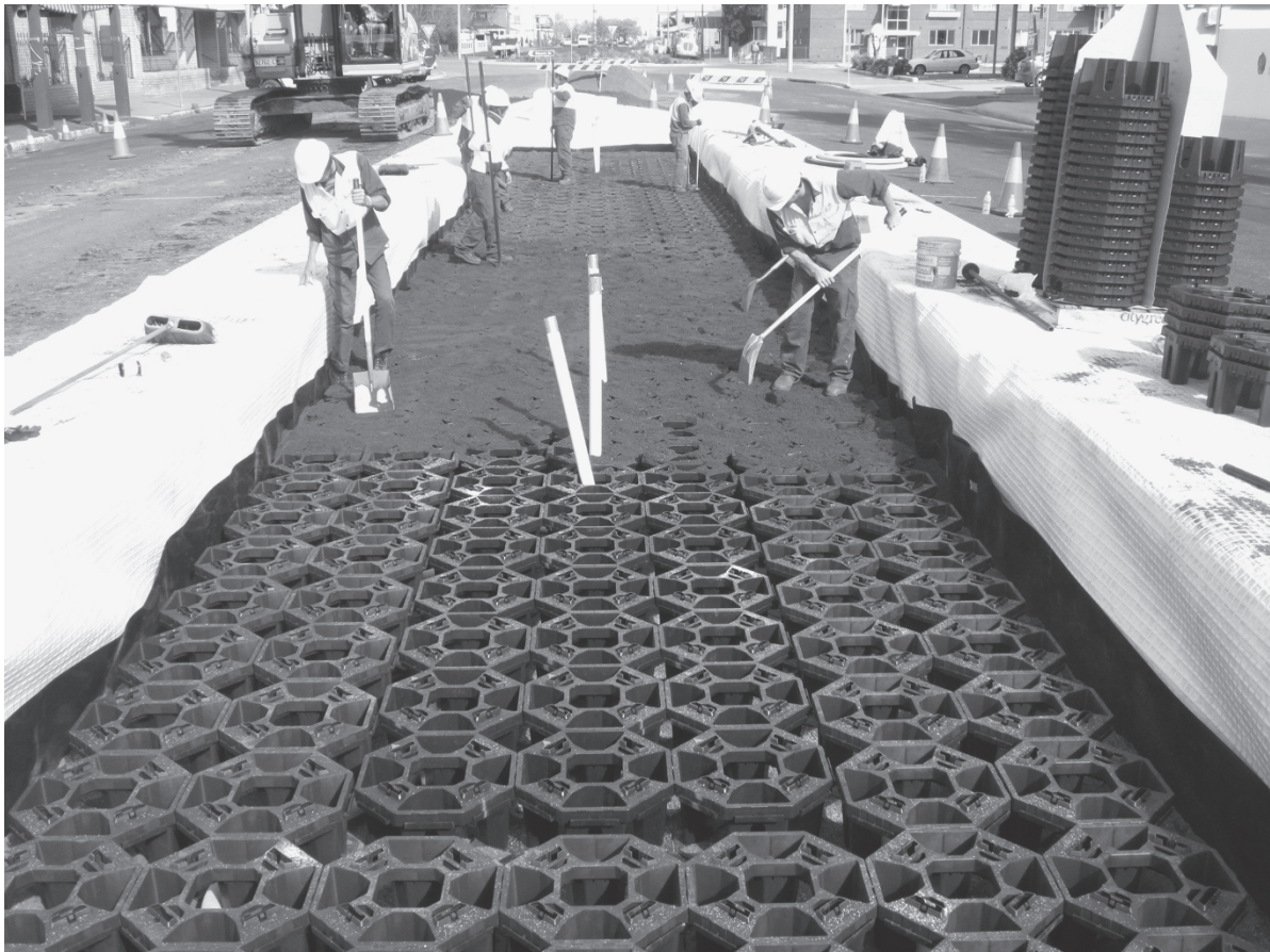
Figure 3.26 “Cells” to support suspended pavement are a relatively recent addition to the toolkit for protecting street trees. Strata Cells, shown here, are designed to stack for efficient shipping (right rear). (Project and Photo: Citygreen.)
