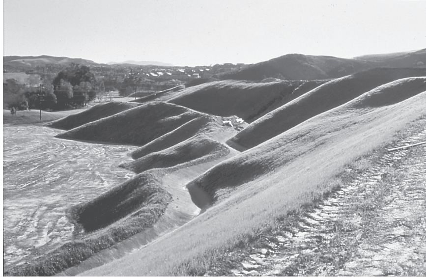
Figure 2.10 Landform grading creates forms that resist erosion by being in equilibrium, and that increase habitat diversity and aesthetic appeal. Lifetime costs of creating and maintaining these forms are less than for conventional grading. (Project and Photo: H. J. Schor.)
