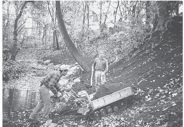
Figure 7.13 Motorized wheelbarrows, like this Honda Power Wagon or the newer Power Carrier, can do heavy work with decreased site impact, as in Sweet Brook’s restoration. (Project: NY DEP. Photo: Dean Cavallaro.)
