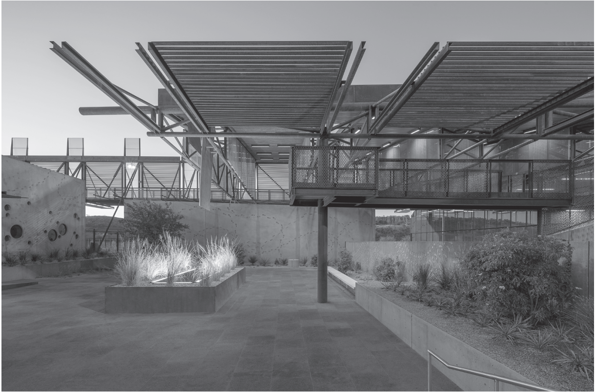
Figure 4.19 Water harvested from roof and landscape is stored for dry-season use at Mariposa Port of Entry, Nogales AZ. A 1-million-gallon tank holds the rainwater. Solar hot water and electricity, as well as recycled materials and native plantings, are other features of this building, one of many commissioned by the General Services Administration. (Project: Chris Winters & Assoc. and Jones Studio. Photo: Bill Timmerman.)
