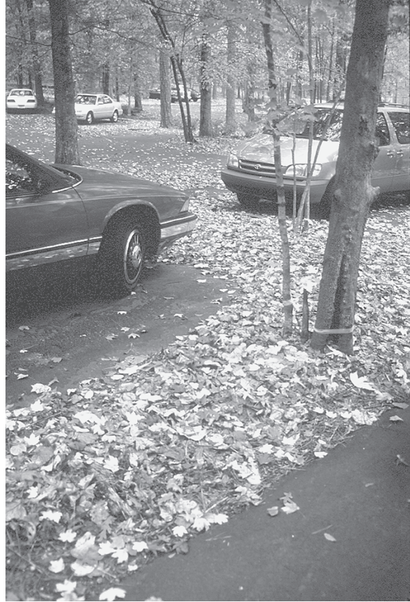
Figure 5.16 Dispersed parking for Simmons headquarters reduced disruption and infiltrates runoff near its source. (Project: Robert Marvin Associates. Photo: Bruce Ferguson.)
