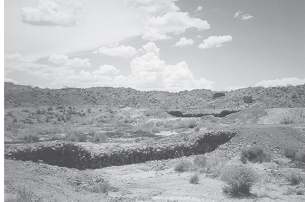
Figure 4.4 More effective than a single massive dam, a series of small check dams stop and infiltrate water throughout a stream or gully. Only the highest floods overflow spillways. (Photo: New Mexico Department of Mining and Minerals.)
