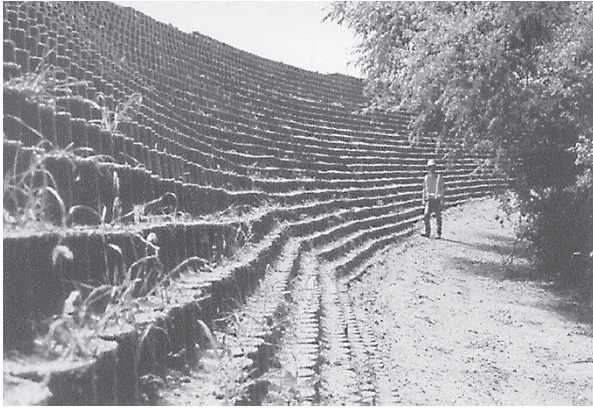
Figure 3.11 Cellular containment materials are flexible honeycombs filled with soil or gravel. A single layer can form a drivable surface; stacked as shown, cells form a greenwall. (Photo: Webtec.)
