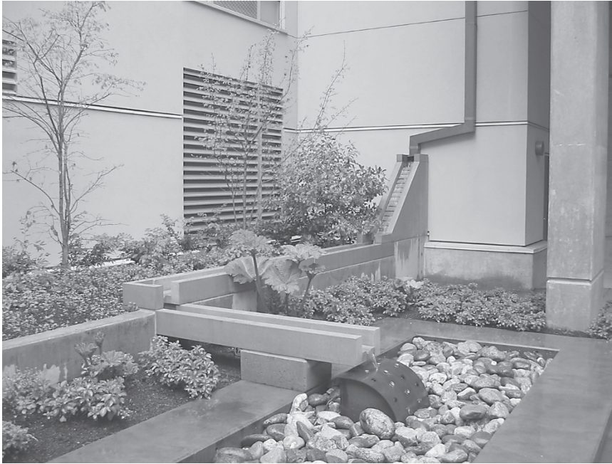
Figure 4.24 The 10th@Hoyt courtyard (Portland OR) makes rainwater visible and artful en route from roof to cistern. (Project: Steve Koch. Photo: Stuart Echols.)
