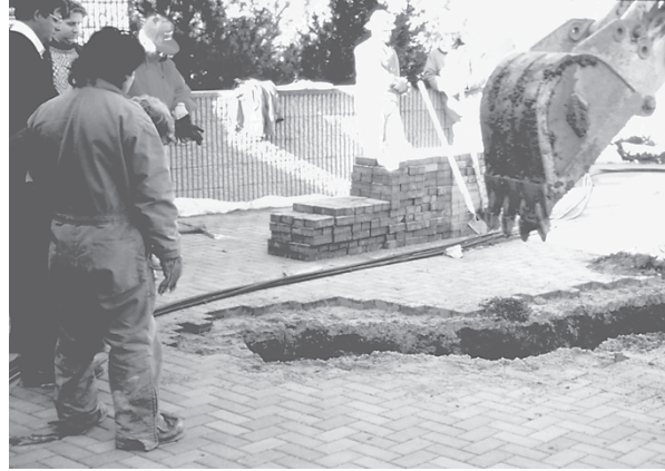
Figure I.9 Interlocking pavers set on sand are easily removed and replaced for utility access, saving energy, cost, and waste. Some pavers also permit water infiltration. (Photo: Courtesy of Interlocking Concrete Pavement Inst. / David R. Smith.)
