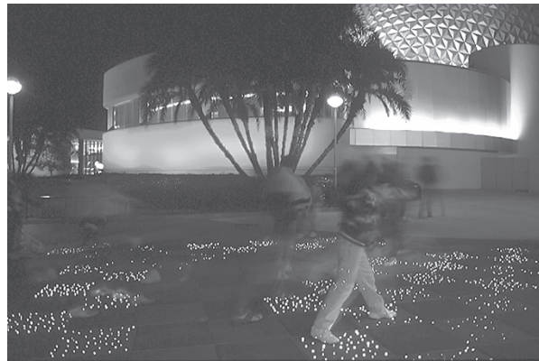
Figure 8.3 End-emitting fiber-optics in Epcot’s sidewalk create a moving, color-shifting bed of stars. Attracting more attention than the floodlights, they use far less energy. (Photo: Kim Sorvig.)
