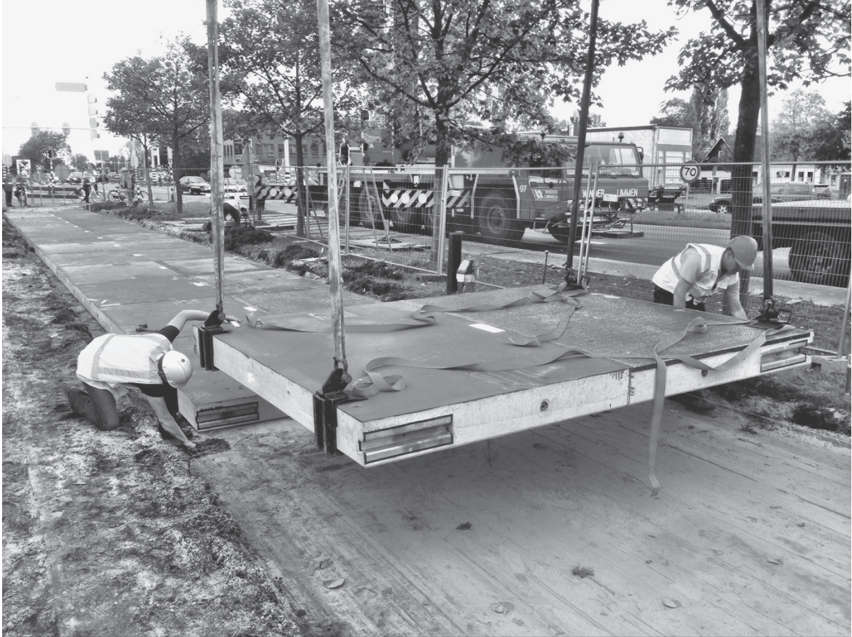
Figure 7.5 Large modular PV panels are placed for a bike and walking path that generates energy in Holland. (Product and Photo: SolaRoad Netherlands [courtesy photo].)
