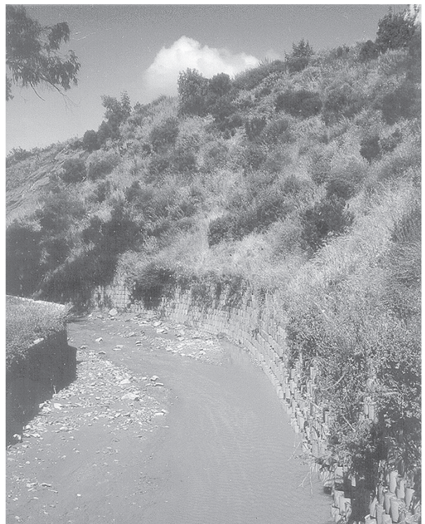
Figure 3.12a, b Greenwalls can reduce the “footprint” or horizontal extent of a high bank by steepening it. This approach protects Crystal Cove State Park (CA) from increased upstream runoff—shown during (a) and after construction (b). (Project: California State Parks, Steve Musillami. Photo: Alan Tang.)
