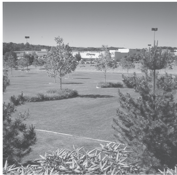
Figure 5.13 Overflow parking at Westfarms Mall uses Grasspave 2 instead of impervious asphalt. (Photo: Invisible Structures.)
