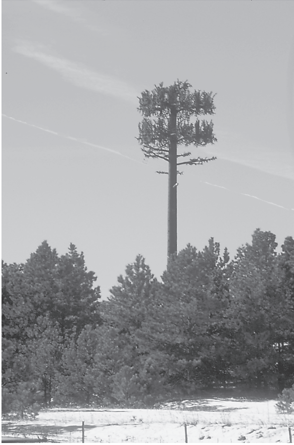
Figure I.II Cell-phone towers, even when disguised as trees, mar the landscape visually and harm wildlife; access roads cause environmental disruption. (Photo: Kim Sorvig.)
