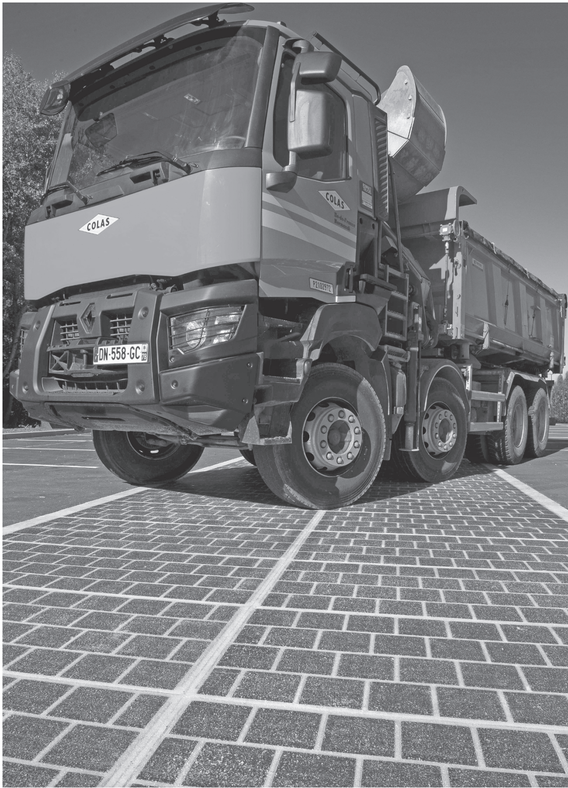
Figure 7.6 Small and thin—but tough—Wattway PV panels install over existing pavement. These were used for France's first solar roadway, at Tourouvre-au-Perche. (Product: Colas. Photo: © COLAS—Joachim Bertrand [courtesy photo].)
