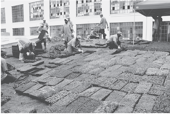
Figure 3.I4 A greenroof ready to plant, showing porous aggregate lightweight planting mix. (Project: Emory Knoll Nursery. Photo: Ed Snodgrass.)
