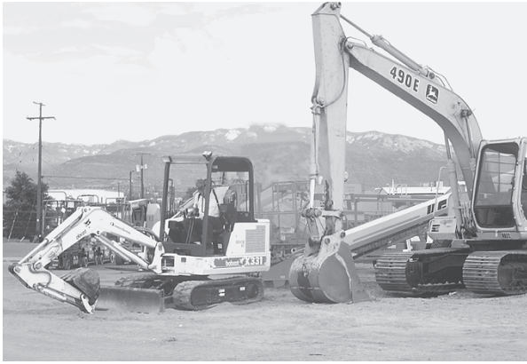
Figure 7.10 Some “heavy equipment” isn’t. The small Bobcat excavator is about seven feet tall by three feet wide. Compared to the larger excavator shown, weight and fuel use are about 10 percent. (Photo: Kim Sorvig.)
