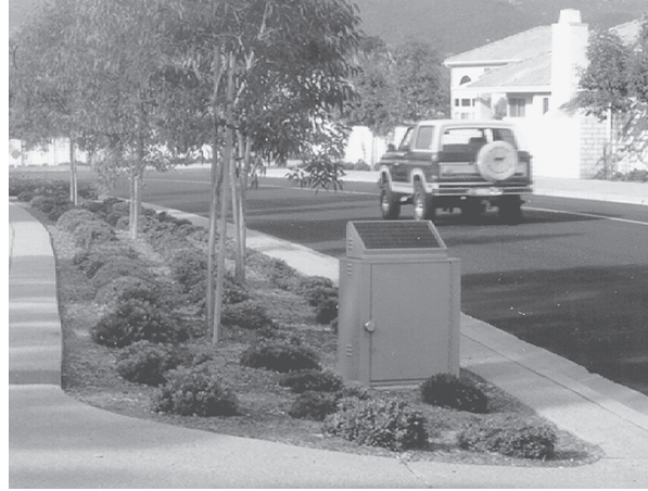
Figure 4.28 An early solar irrigation controller with an inverter to provide 110V AC power to standard valves. (Photo: Photocomm/Golden Genesis Co.)
