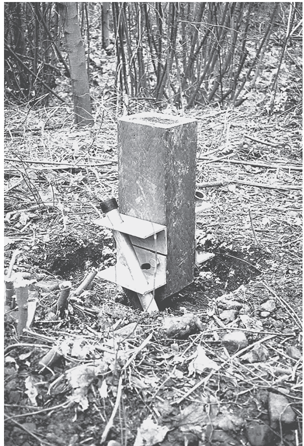
Figure 6.18 Recycled plastic lumber piers support decks along the Upper Charles River near Boston. Metal “pinned foundations” cause almost no site disruption and can be removed or adjusted easily. (Project and Photo: Carol R. Johnson and Associates.)
