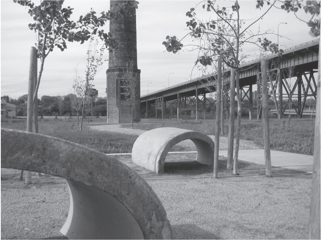
Figure 0.8 The Menomenee Valley Redevelopment produced park and property development from a brownfield, recycling 50,000 cubic yards of crushed concrete from reconstruction of I-94, and reused on-site features. (Project: Wenk Assoc. Photo: Nancy Aten.)
