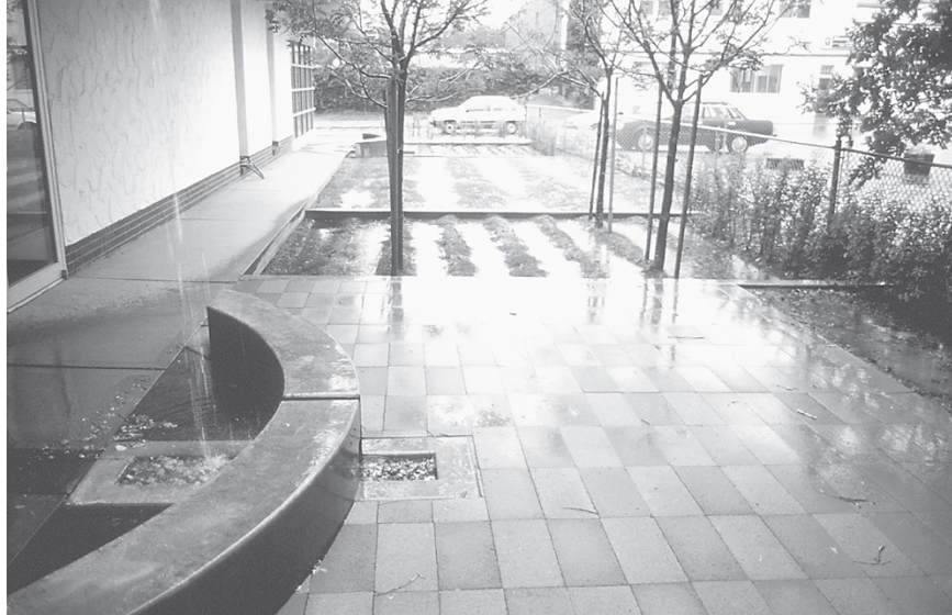
Figure 4.22 Rainwater from a roof drain is caught in a gravel basin and routed to furrows in the garden at the Denver offices of designer Bill Wenk. (Project and Photo: Bill Wenk.)
