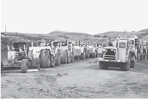
Figure I.I4 Staging areas (this one is for a fairly small road project) can permanently damage an expanse larger than the site of actual work. (Photo: Kim Sorvig.)
