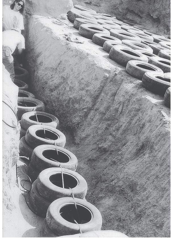
Figure 6.16 Check dams reuse waste tires to stabilize an arroyo in Arizona. Tires in the trench form a footing for the dam at the upper level. (Project and Photo: Stuart Hoenig and Joshua Minyard.)
