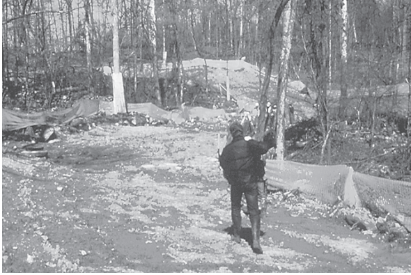
Figure I.8 This easement, in Loudon County VA, is less than half as wide as the utility's standard. Note the site protection fence. (Project: Park Authority, HOH Associates, and Rhodeside and Harwell. Photo: Doug Hays.)
