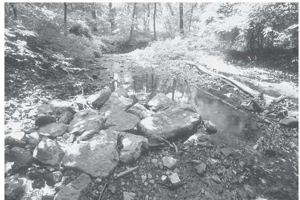
Figure 4.13 Stone deflector in restored Wheaton Branch unobtrusively guards the stream bank from floods. (Project: Washington Council of Governments. Photo: Walt Callahan.)
