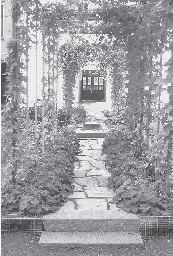
Figure 6.4 Salvaged during demolition, roof tiles form curbs and gutters, and fill gabion-like planted walls in this urban garden in Oslo, Norway. Crushed tile surfaces paths, and serves as concrete aggregate. Stone, too, is second hand. (Project: Snohetta Landskapsarkitekter. Photo: Rainer Stange.)
