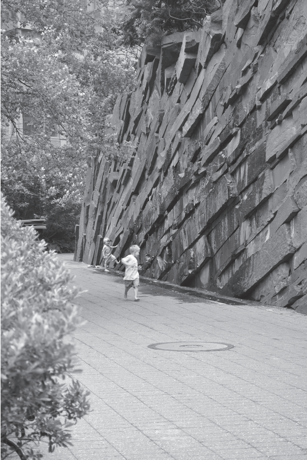
Figure 0.13 This water/ice wall (Teardrop Park, Battery Park City) is an urban amenity constructed from quarried stone, naturalistic without being literally imitative. Besides water play, its surface offers habitat that no monolithic concrete wall could. ( Project and Photo: Michael van Valkenburgh Assocs. )
