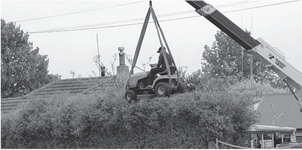
Figure II.2 A real “landscape fail”—crane and mower hedge trimming—fortunately without injury. ( Project: subject insisted on anonymity. Photo: Bart Dinger, Hamilton NZ. )
