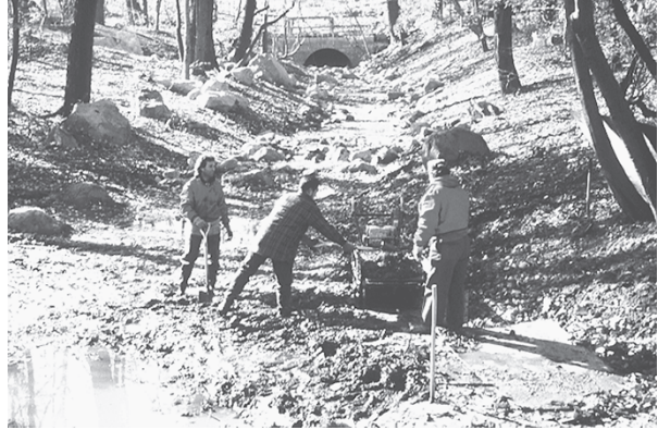
Figure 4.14 Tons of accumulated sediment were removed from Sweet Brook and used to fertilize the restored banks. (Project: New York City Department of Environmental Protection. Photo: Dean Cavallaro.)
