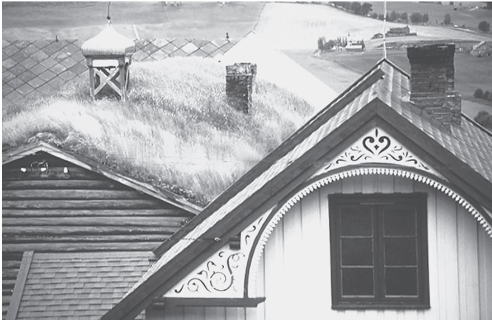
Figure 3.13 Ecoroofs are an update on traditional sod roofs—an example of revisiting past technologies to meet sustainability goals. (Photo: Kim Sorvig.)
