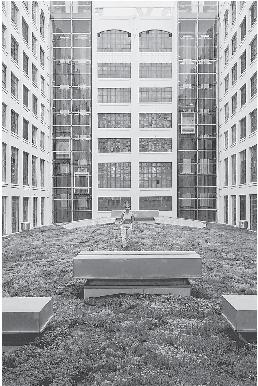
Figure 3.18 Montgomery Park Business Center (Baltimore) boasts a thriving light-weight greenroof. (Project: Katrin Scholz-Barth. Photo: Kai-Henrik Barth.)
