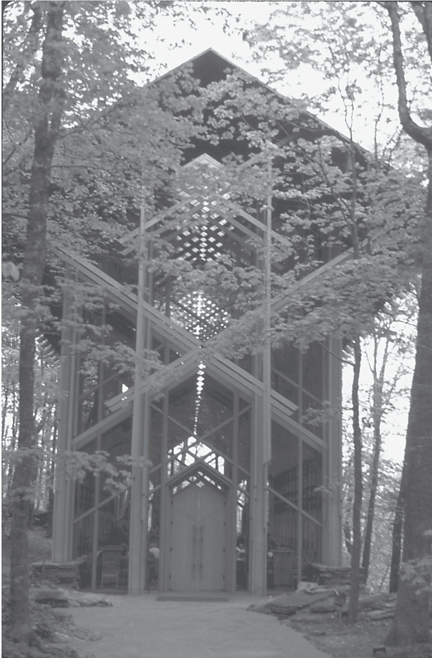
Figure I.16 Thorncrown Chapel is a national treasure, in part because nonmechanized construction preserved its relationship to the woods. (Project: E. Fay Jones. Photo: Stephen Schreiber.)
