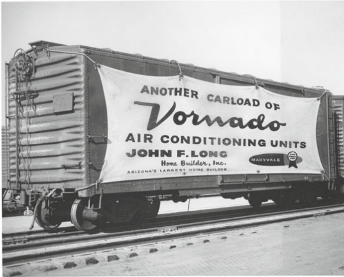
Figure 3.1. Train car delivery of home air-conditioning units. (Source: John F. Long)
