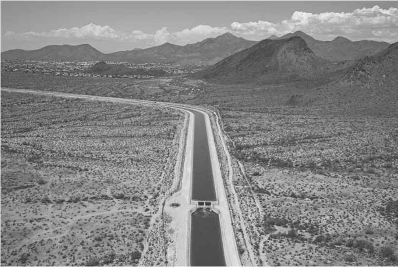
Figure 2.3. The Central Arizona Project (CAP) is designed to bring approximately 1.5 million acre-feet of Colorado River water annually to Pima, Pinal, and Maricopa Counties. (© Shutterstock: Tim Roberts Photography)
