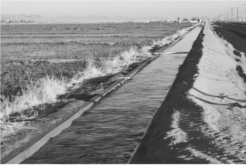
Figure 2.2. Water being delivered for irrigated agriculture in central Arizona. (© Shutterstock: Jim Parkin)
