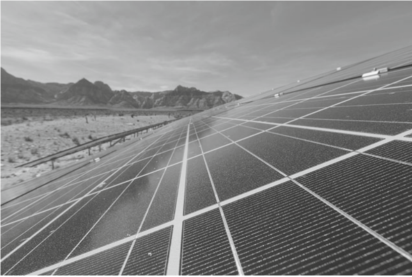
Figure 3.2. Solar panels in the desert. (© Shutterstock: Andrei Orlov)
