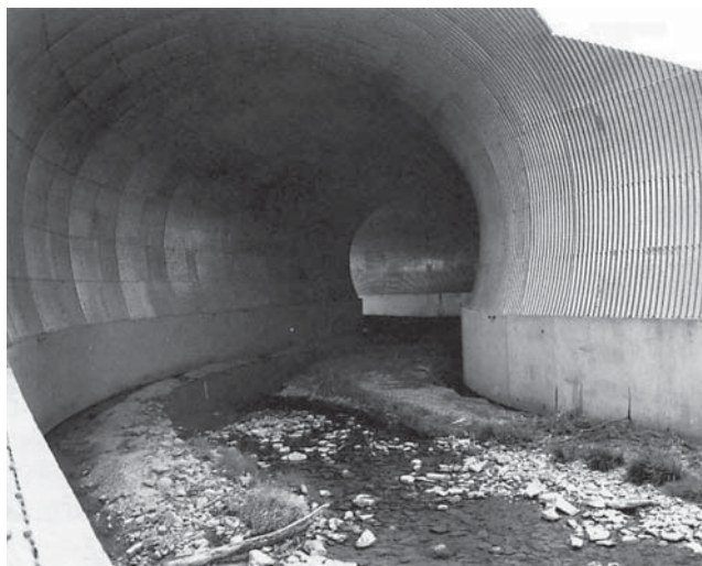
FIGURE 24.2 Deer crossing. (Courtesy of CONTECH Construction Products Inc., Olde West Chester, OH, reprinted from sitesolutionsmag.com.)
