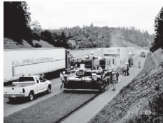
Recycling with traffic in adjacent lane
