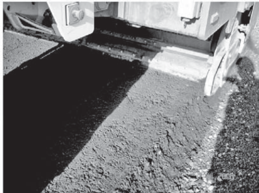
300 mm FDR with cement slurry with 5.8% cement
