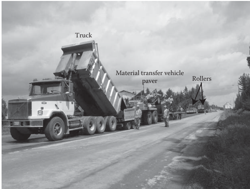
FIGURE 16.12 Different equipment used in hot mix asphalt paving. (Courtesy of Carolina Carbo, Road Recycling Council.)
