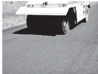
Finish rolling with rubber tired roller
