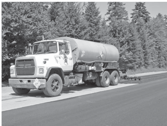
FIGURE 16.11 Application of tack coat. (Courtesy of Carolina Carbo, Road Recycling Council.)
