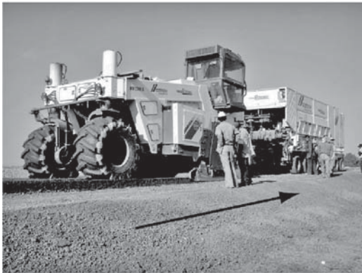
FDR using WR 2500S recycler and WM 100 cement slurry equipment
