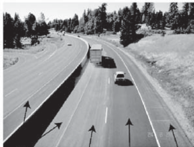
Recycled shoulder Recycled no.1 lane Mill and fill no.2 lane Recycled shoulder
