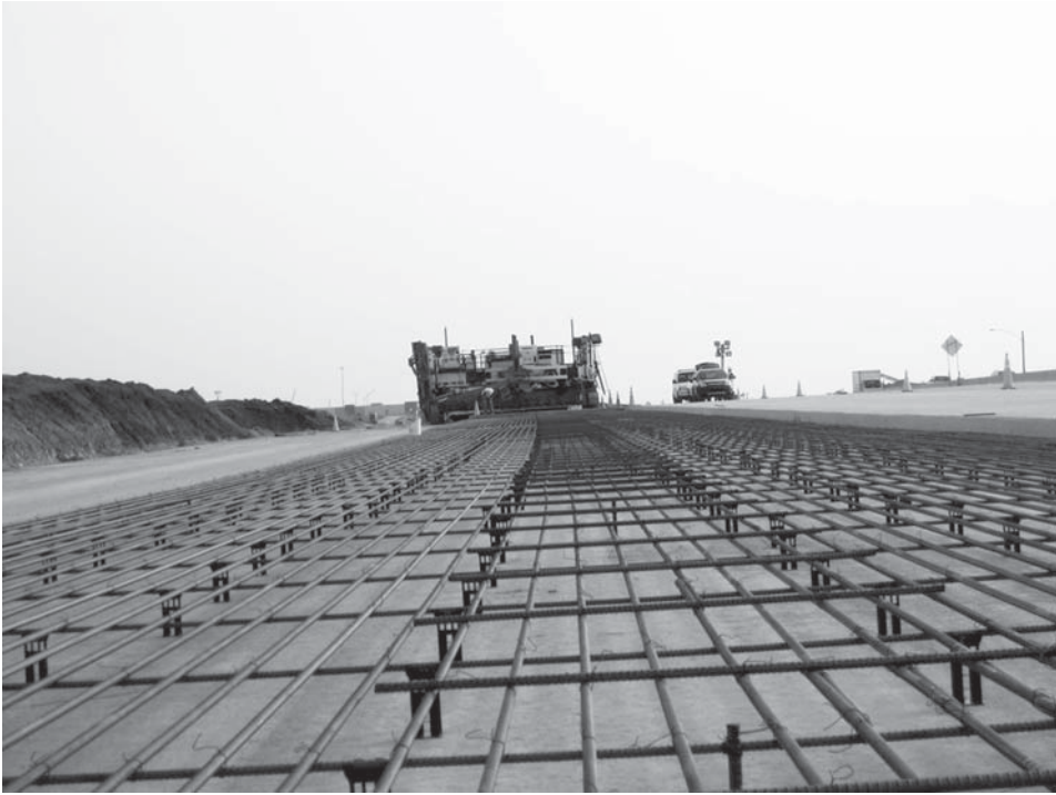
FIGURE 15.23 CRCP under construction.
