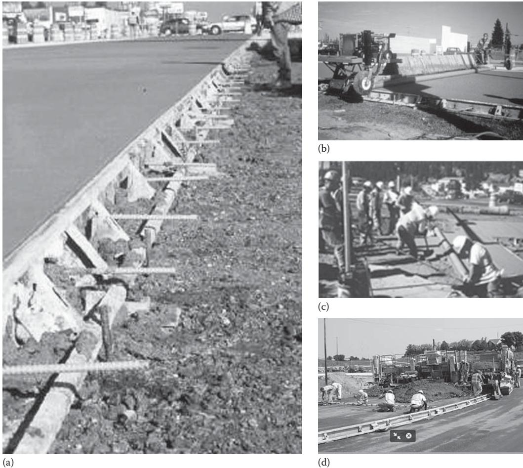
FIGURE 17.9 Typical fixed form construction operations. (ACPA)
