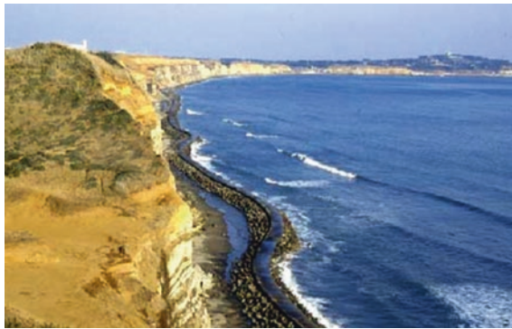
Fig. 2.38 Cliff recession halted by a shore wall at Byobugaura on the east coast of Japan. © Geostudies
