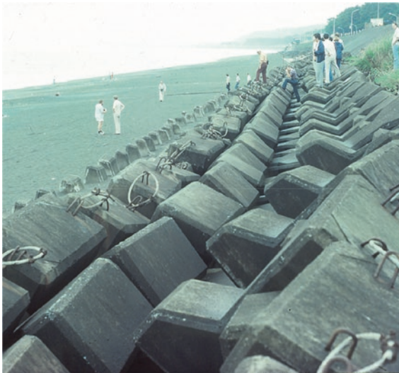
Fig. 7.2 Concrete blocks protecting a cliff in Japan. © Geostudies
