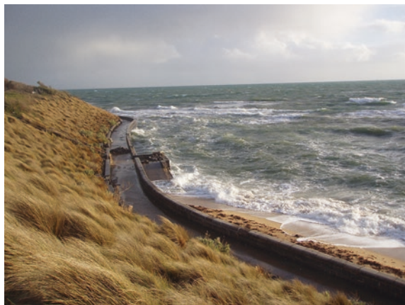
Fig. 5.3 A former cliff stabilised as a sloping grassy bluff at Quiet Corner, Victoria, Australia. Most of the natural cliff in the coastal suburb of Bayside, Melbourne, have been treated in this way: Red Bluff (Fig. 6.2) is one of the few short stretches of natural cliff on the coast of Port Phillip Bay that have survived. © Geostudies
