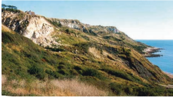
Fig. 3.1 Irregular topography produced by mass movement on the coast at White Nothe, Ringstead, Dorset. © Geostudies
