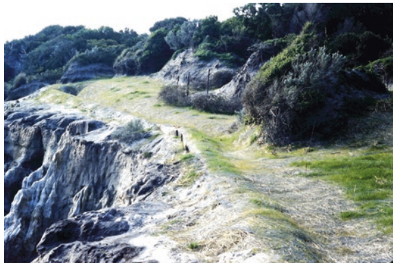
Fig. 3.10 Cliff-top drain inserted to intercept runoff at Black Rock Point, Victoria, Australia. © Geostudies
