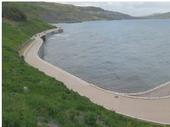
Fig. 7.8 The stabilised coast at Church Cliffs, Lyme Regis, Dorset, in 2015. © Geostudies
