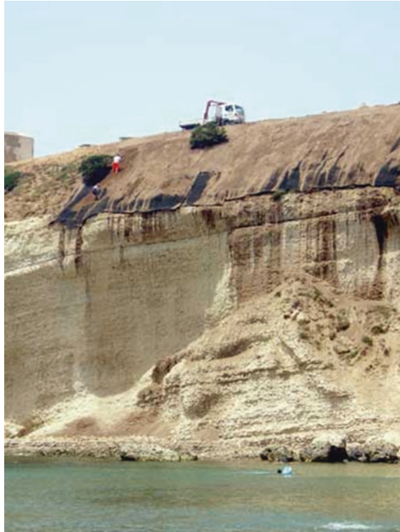
Fig. 7.9 Stabilisation of a coastal slope in sandy clay at Santa Catterina di Pittinuri on the west coast of Sardinia.
