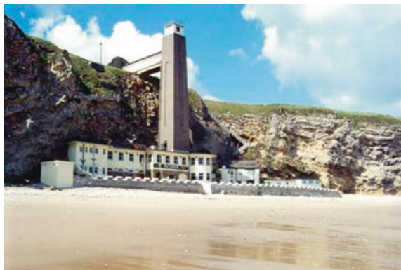
Fig. 3.30 Building against a cliff on the Durham coast. © Geostudies
