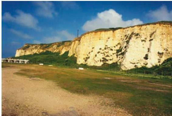
Fig. 2.39 The Chalk cliff behind Newhaven harbour in Sussex has been modified following harbour construction. A slope has formed on the capping of Eocene clays, above an apron of down-washed sediment. The formerly vertical cliff is thus developing a convex-over-concave profile. © Geostudies
