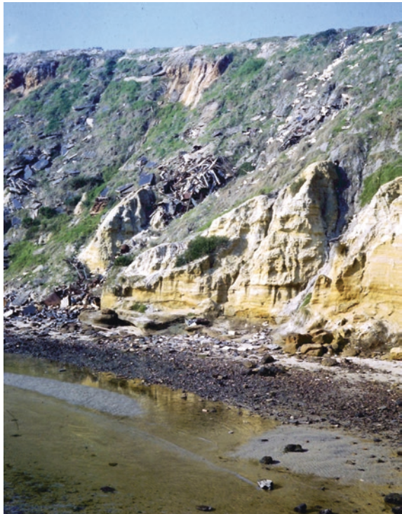
Fig. 3.36 Rubble waste dumped on the cliff at Red Bluff, Victoria, Australia. © Geostudies
