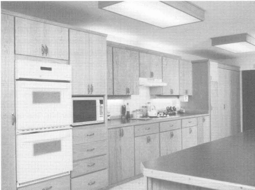
Simple wood veneer particleboard sheets with wood edge tape look great and are an inexpensive door option for those large projects.
