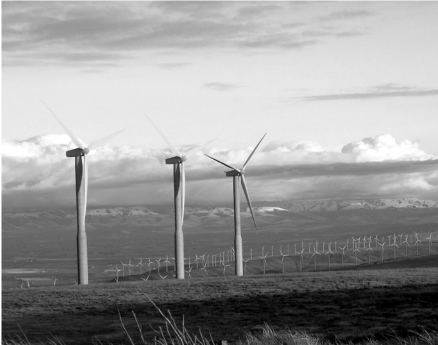
Fig. 1 Modern, three-bladed, upwind-type of HAWT on a wind farm (In this case, the wind is blowing from right to left)
