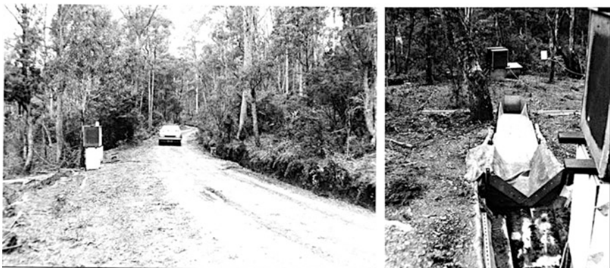
Fig. 4.4 Road runoff. The photograph to the left is a stretch of forest road. The box is a streamflow measurement structure mounted on a culvert. The photograph on the right shows the measurement weir. Water passing out of this was distributed over the slope. A second measurement weir downslope estimated slope infiltration. The work is detailed in Bren and Leitch (1985)
