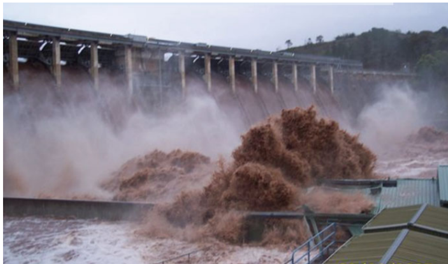
Fig. 8.13 Glenmaggie weir passing a peak flow of around 260,000 \text{ ML day}^{-1} on June 28th, 2007, about 6 months after the catchment was burnt. This was in excess of expected flow levels for the given rainfall. The surging in the foreground is water impacting on a power station. The colour of the water shows severe erosion (Photograph courtesy of Joe Matthews and Southern Rural Water)
