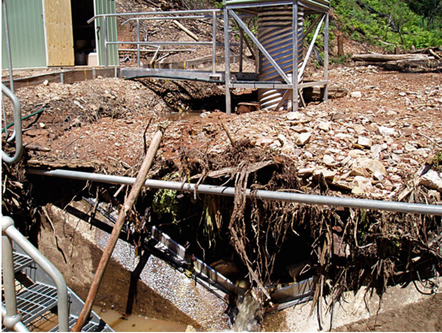
Fig. 8.3 Soil erosion at Croppers Creek about 1 year after burning. Such erosion tended to be associated with “spike flows”
