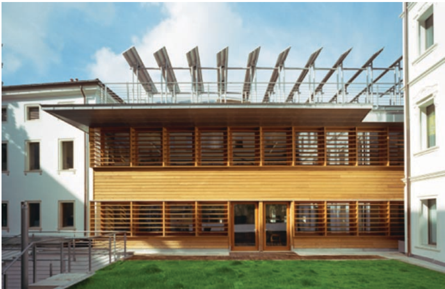
Fig. 4.4.1 Banca Etica headquarters in Padova, designed and constructed according to bio-ecological architecture principles (Courtesy: Banca Etica) (see Color Plates )
