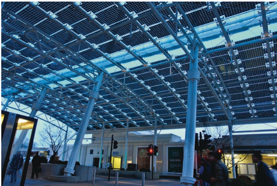
Fig. 6.1.5.1 Photovoltaic array at the station (Courtesy: ICLEI)
