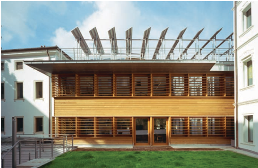
Fig. 4.4.1 Banca Etica headquarters in Padova, designed and constructed according to bio-ecological architecture principles
