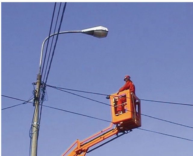
Fig. 6.2.2.1 Light bulb replacement in progress (see Color Plates )
