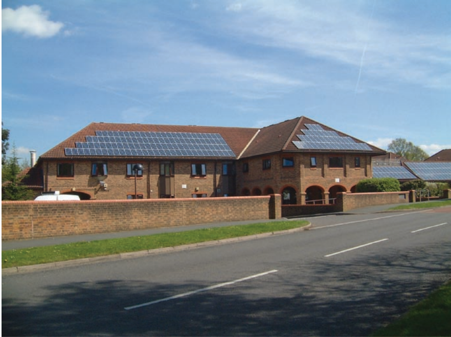
Fig. 6.1.5.2 Brockhill retirement village with a huge photovoltaic (PV) array on the roof and a residential Combined Heat and Power (CHP) system (see Color Plates )
