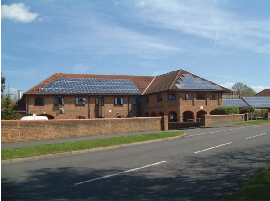
Fig. 6.1.5.2 Brockhill retirement village with a huge photovoltaic (PV) array on the roof and a residential Combined Heat and Power (CHP) system
