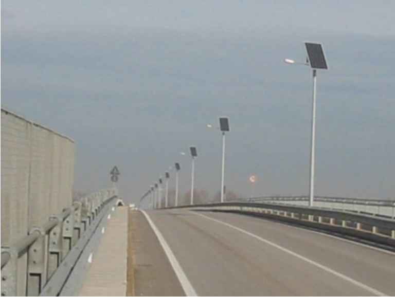
Fig. 6.2.5.1 Lighting on the bridge of the Po River
