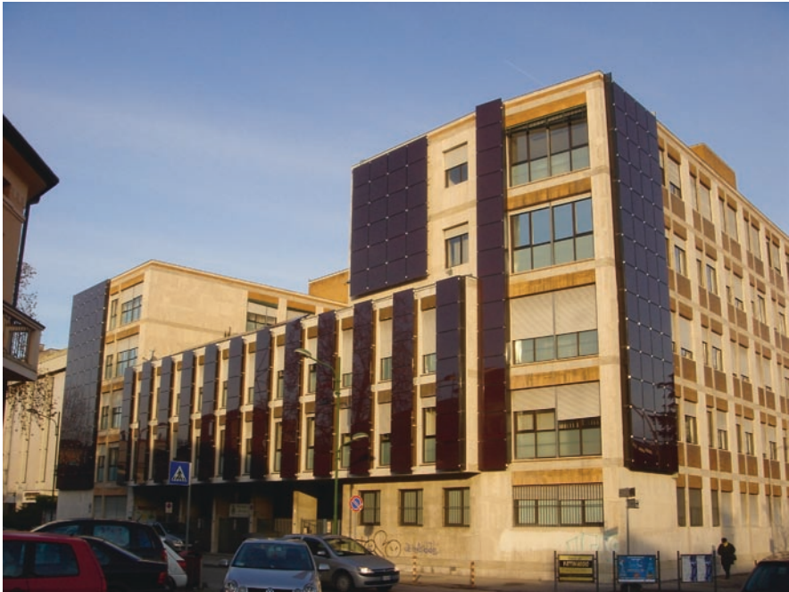
Fig. 6.2.5.3 Photovoltaic facade of the Province of Rovigo office building (see Color Plates )
