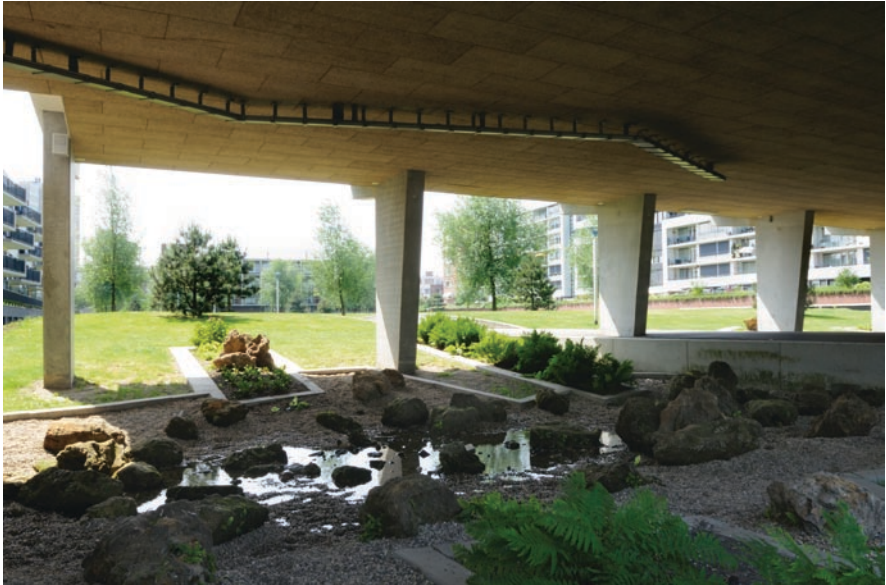
Fig. 2.1.1 Adaptation measure: a rainwater infiltration area below a building in Tilburg. A wadi ( Arabic word meaning dry riverbed that contains water only during times of heavy rain ) offers a way to deal with heavy rainfalls by buffering overflowing water and reducing the risk of flooding. In addition the wadi cools the area and offers a nice environment for plants, animals and insects (Photographer: Maartje Ansems)
