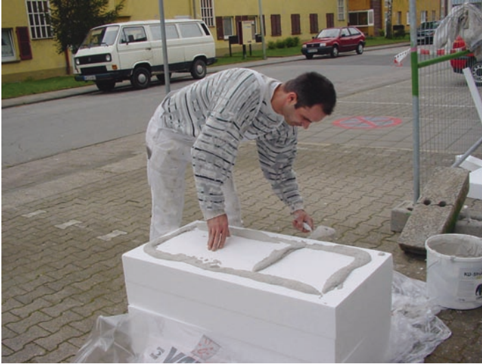
Fig. 6.3.4.3 Craftsman preparing wall insulation
