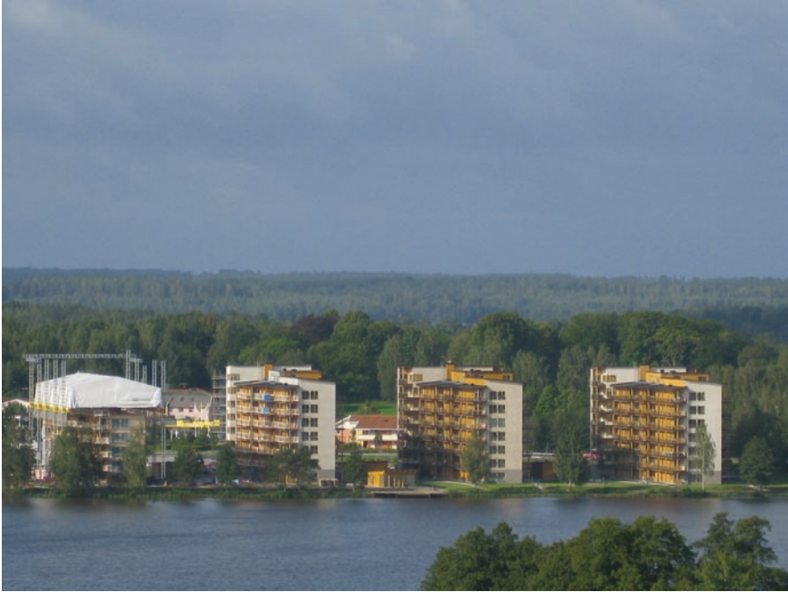
Fig. 6.1.1.2 New concepts in development – eight-storey high wooden buildings constructed within the CONCERTO SESAC project (Photographer: Anders Nordenskiöld) (see Color Plates )
