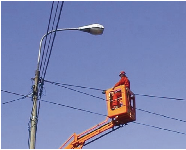
Fig. 6.2.2.1 Light bulb replacement in progress
