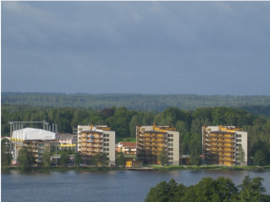
Fig. 6.1.1.2 New concepts in development – eight-storey high wooden buildings constructed within the CONCERTO SESAC project (Photographer: Anders Nordenskiöld)
