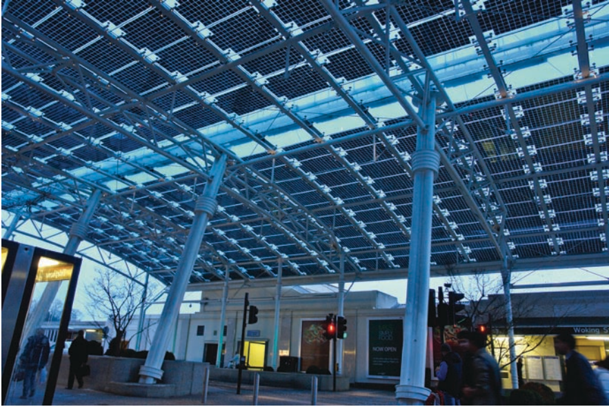
Fig. 6.1.5.1 Photovoltaic array at the station (Courtesy: ICLEI) (see Color Plates )
