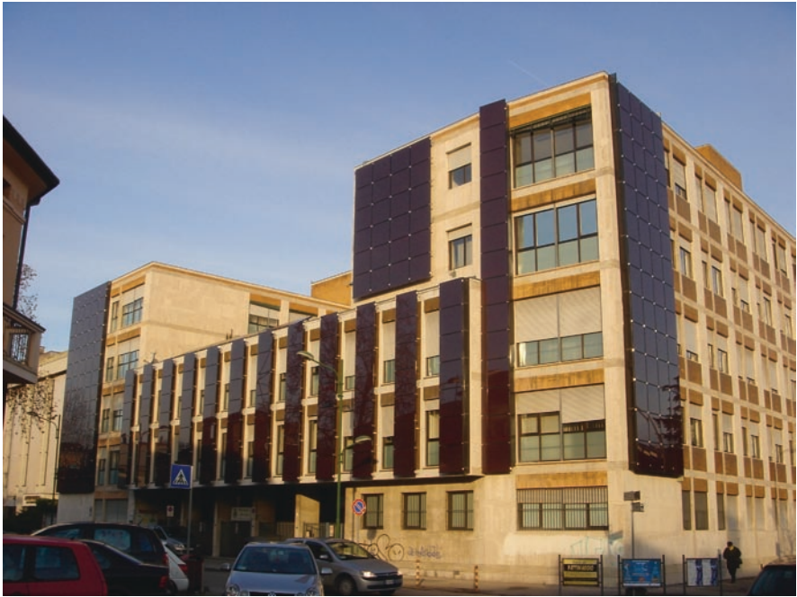
Fig. 6.2.5.3 Photovoltaic facade of the Province of Rovigo office building
