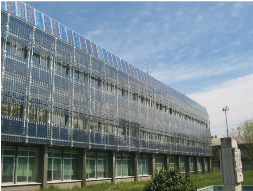
Fig. 6.2.5.2 Photovoltaic facade of the secondary school ITIS (see Color Plates )
