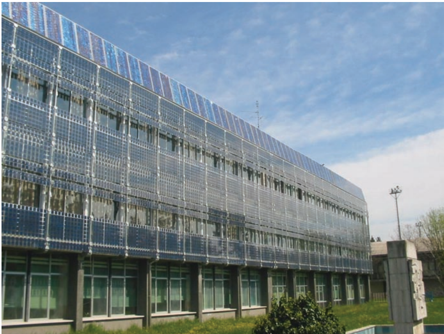
Fig. 6.2.5.2 Photovoltaic facade of the secondary school ITIS
