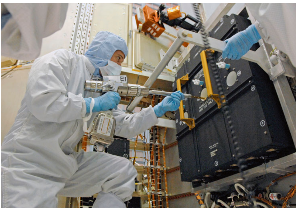
Michael Good (STS-125) practices installing a battery module into the Hubble High Fidelity Mechanical Simulator, in the cleanroom at NASA's Goddard Space Flight Center.
