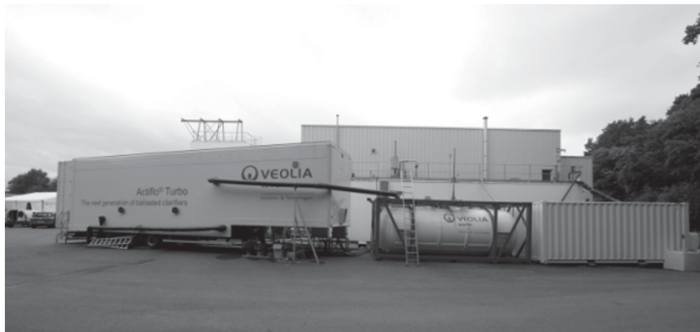
Figure 4. The Pilot plant.
