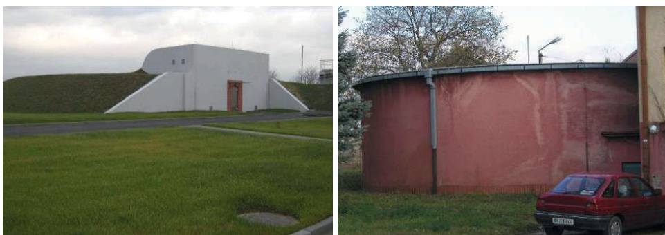
Figure 4. Reconstruction of WTP Lednice – accumulation tank before and after the reconstruction.
