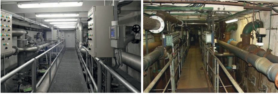
Figure 5. Reconstruction of WTP Lednice – pipelines and equipments before and after.
