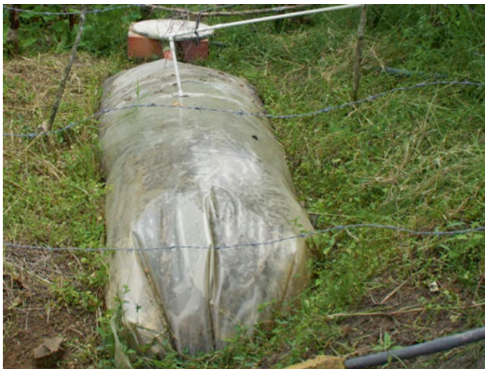
Photo 22 Waste water from the kitchen, the clothes washer and the machine for pulping fresh coffee beans is directed to this biodigester
