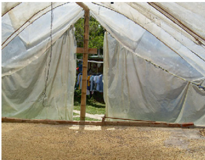
Photo 7 “Guadua” provides the support structure of the plastic canopy for drying the coffee beans, the bagasse and the stems of mulberry and Tithonia
