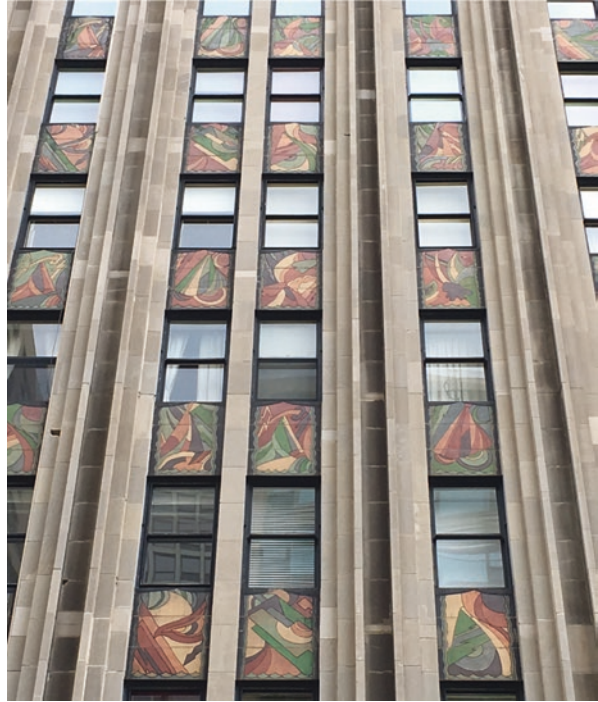
Fig. 15.2 These, too, are spandrels. Art deco terra cotta spandrels on the Powhatan building in Chicago. Photograph by Mary Nitsch
