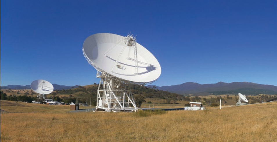
Figure 4.8. Dishes of the Canberra Deep Space Network pointed at Mars. In this photo, taken on November 18, 2013, two 34-meter dishes (DSS-34 at center and DSS-45 at right) were listening to signals from the MAVEN orbiter as it arrived at Mars. At the same time, at left, the 70-meter DSS-43 simultaneously received data from Mars Odyssey and Mars Reconnaissance Orbiter. Photo courtesy Glen Nagle, Canberra Deep Space Communication Complex.
