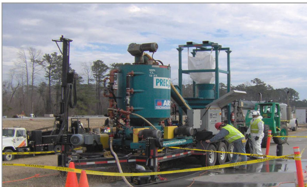
Figure 11.12. Potassium permanganate mixing and pneumatic injection (in the background).
