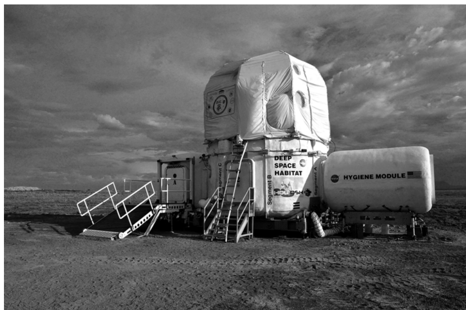
Fig. 9.12 The outdoor version of NASA's Deep Space Habitat, with a student-built "penthouse" on top. The two-story living areas are flanked by a hygiene module to the right (Image courtesy of NASA/JSC)
