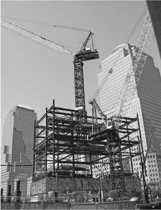
FIGURE 2.43 A luffing jib tower crane on a climbing base sitting within the framework of Freedom Tower at the World Trade Center site. ( Mathieu Chaudanson. )
