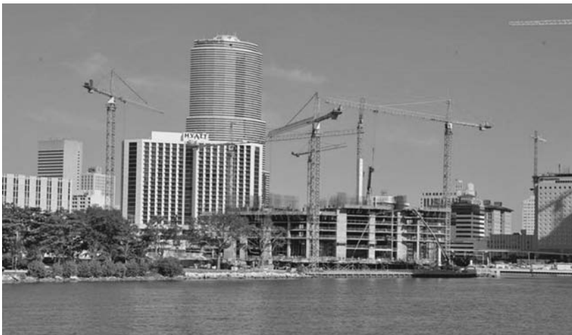
FIGURE 2.38 Overlapping hammerhead tower cranes must be offset in elevation to allow overswing so that there is full hook coverage of the site. (Morrow Equipment Company.)
