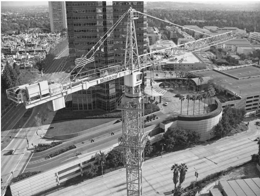
FIGURE 2.32 A saddle jib tower crane in a small U.S. city. All of the key components are visible including a climbing frame. ( Morrow Equipment Corp. )
