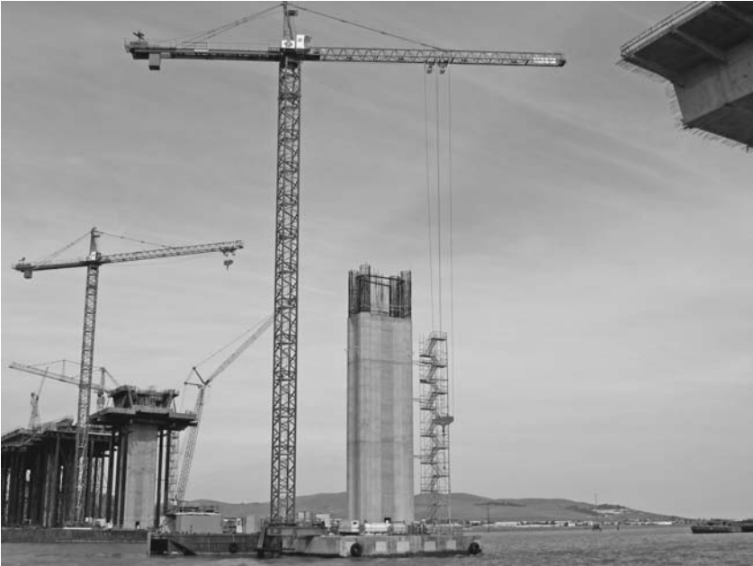
FIGURE 6.6 A freestanding saddle-jib tower crane supported on a cantilevered steel base frame. The base frame must be designed to resist in-service and out-of-service loads and must be stiff enough to keep deflection to a minimum. The high mast and marine location indicate that out-of-service storm wind is likely the controlling design load. (Manitowoc Corporation Inc.)
