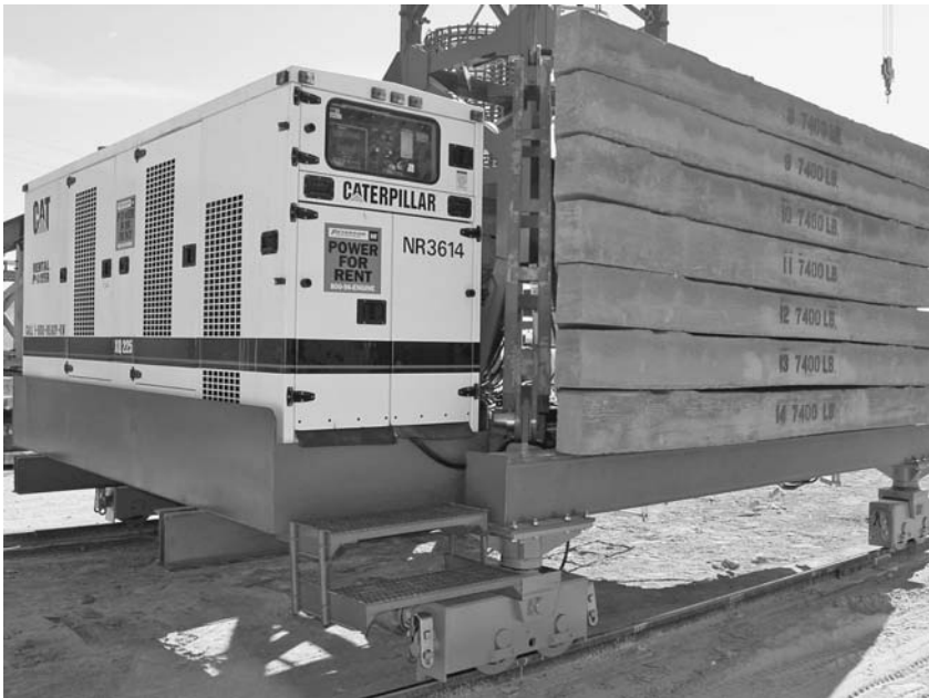
FIGURE 6.39 Bogie, wheels, and rail support for a tower crane on a chassis base. (Manitowoc Corporation Inc.)
