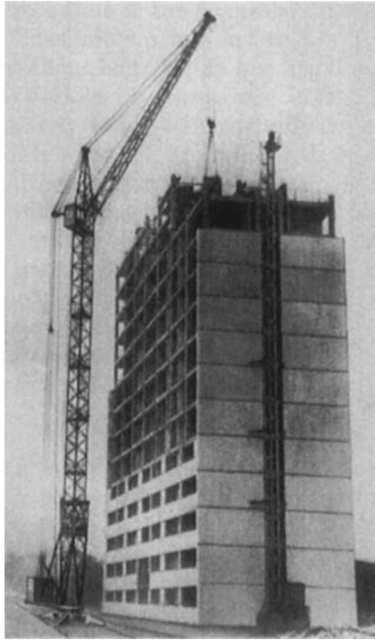
FIGURE 2.34 Luffing jib tower crane built in the former Soviet Union. This rail-mounted crane slews at the bottom. (VNIISTROIDORMASH.)
