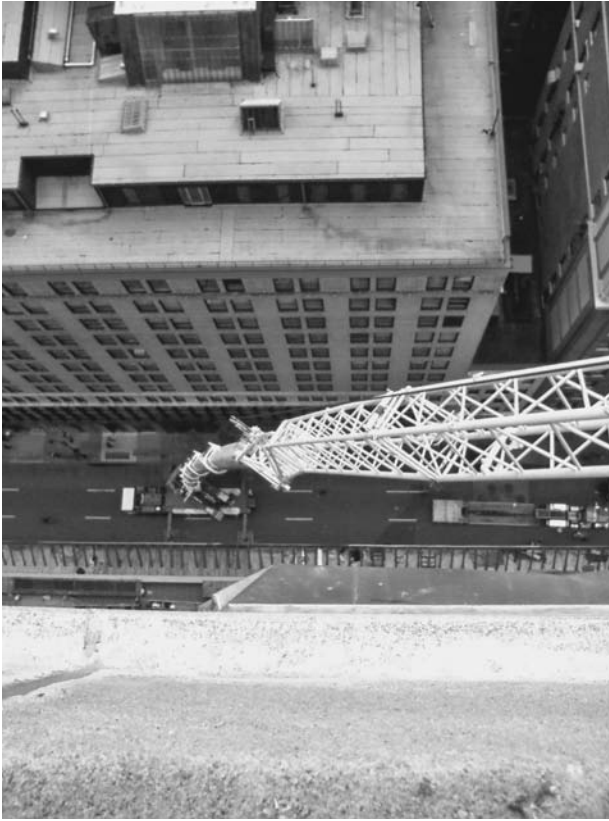
FIGURE 5.12 A view looking down from a roof setback on the Empire State Building to a long-boom telescopic crane on the street below. Deflection can substantially affect the geometry on such machines. ( Mathieu Chaudanson. )
