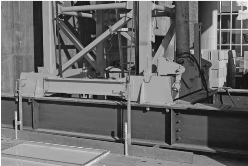
FIGURE 6.30 Climbing base for an internal tower crane provides support for the crane weight during operation. A similar frame at a higher floor supports the climbing ladder . These frames are also used for wedging. There is a subframe below the climbing base that adapts it to the particular building. ( Manitowoc Corporation Inc. )
