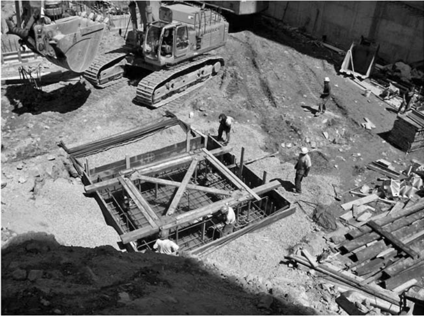
FIGURE 6.14 Template for setting tower-crane anchor bolts. Though well suited for anchor bolts, a template like this must be used with great care for anchor stools as there is no satisfactory means of adjustment after the footing is poured. The footing mass will be supplemented by rock anchors. ( Lawrence K. Shapiro. )
