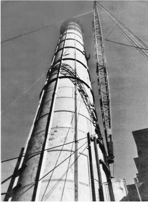
FIGURE 1.19 A 125-ft (38-m) Chicago boom mounted on a steel stack at a Consolidated Edison Company plant in New York City during alterations. Mounting provisions and installation were designed by one of the authors. (Lawrence K. Shapiro.)
