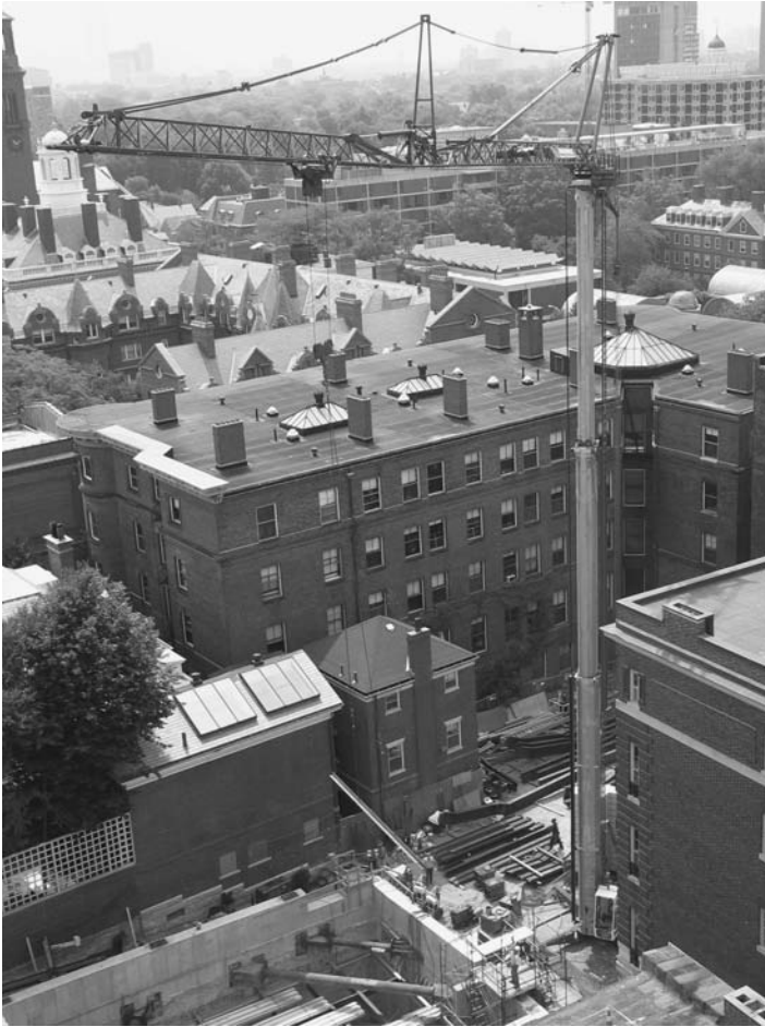
FIGURE 2.35 Self-erecting tower crane with a telescoping mast and articulating jib. The crane is bottom slewing and stabilized by counterweights. ( Morrow Equipment Corp. )
