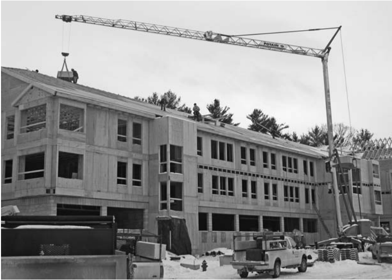
FIGURE 2.44 Small self-erecting tower crane for light construction. The crane is self-contained on a trailer that is towed to the site. ( Manitowoc Company, Inc. )
