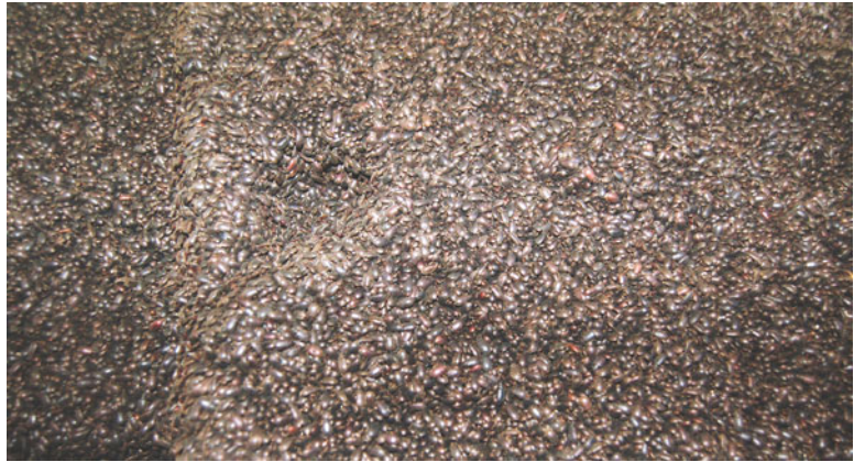
Fig. 11.2 Aggregated L. tristis beetles on the wall of a residential building
