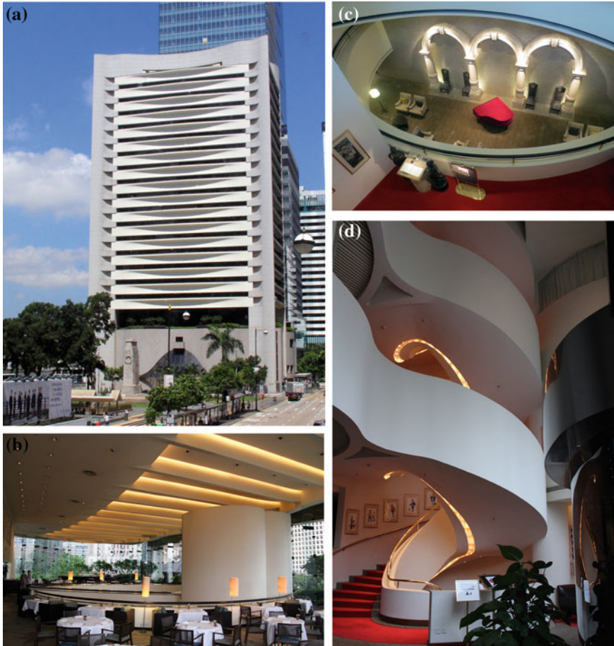
Fig. 7.6 Hong Kong Club, 1984. a The elevation reflects the structural features. b Beams are natural decoration in the dining hall. c The old portico is left as decoration. d Staircase, the curve is signature of Seidler's design
