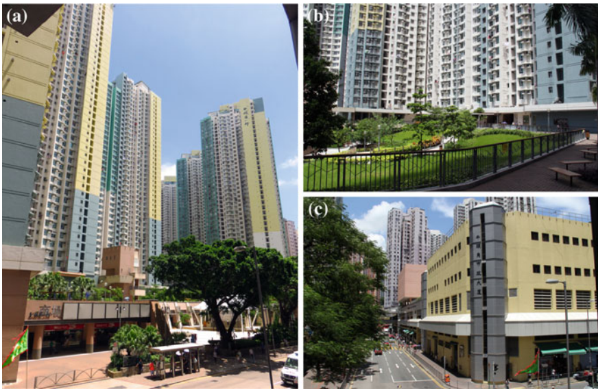
Fig. 2.10 Upper Ngau Tau Kok Estate, 2012. a Housing blocks of 50 stories. b More delicate landscape design closing to the housing entrance. c Market in the estate
