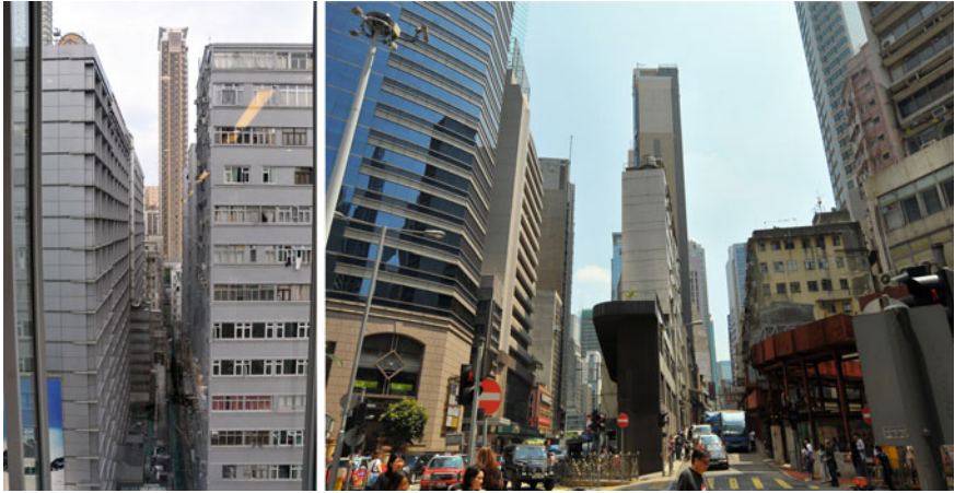
Fig. 4.10 Buildings were continuously redeveloped on the street grid of 19th century
