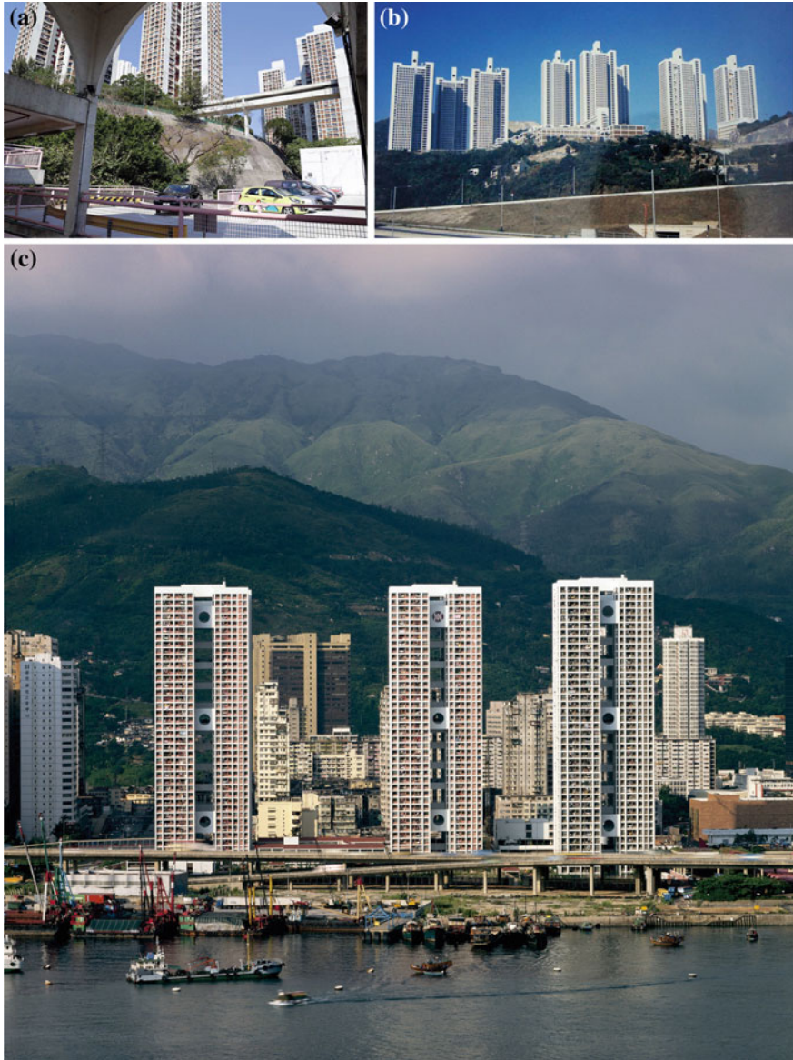
Fig. 2.7 Housing Society's projects designed by Palmer & Turner. a, b Sui Wo Court, 1980. Under the car park is the wet market and shopping arcade. c Clague Garden Estate, 1988. Courtesy of Hong Kong Housing Society
