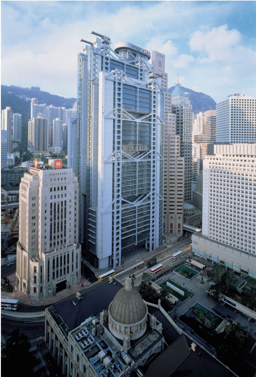
Fig. 7.10 HSBC Bank headquarters completed in 1985. Courtesy of HSBC Asia Pacific Archives
