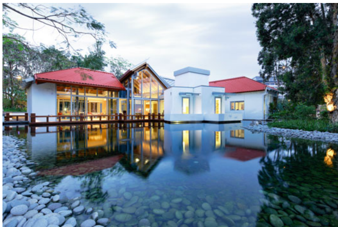
Fig. 7.19 Maggie's Cancer Caring Centre in Hong Kong, 2013. Every component is “non-standard”, which made the construction difficult. Thanks to the BIM system, the size, location and joints could be coordinated in the construction. Courtesy of Ronald Lu & Partners
