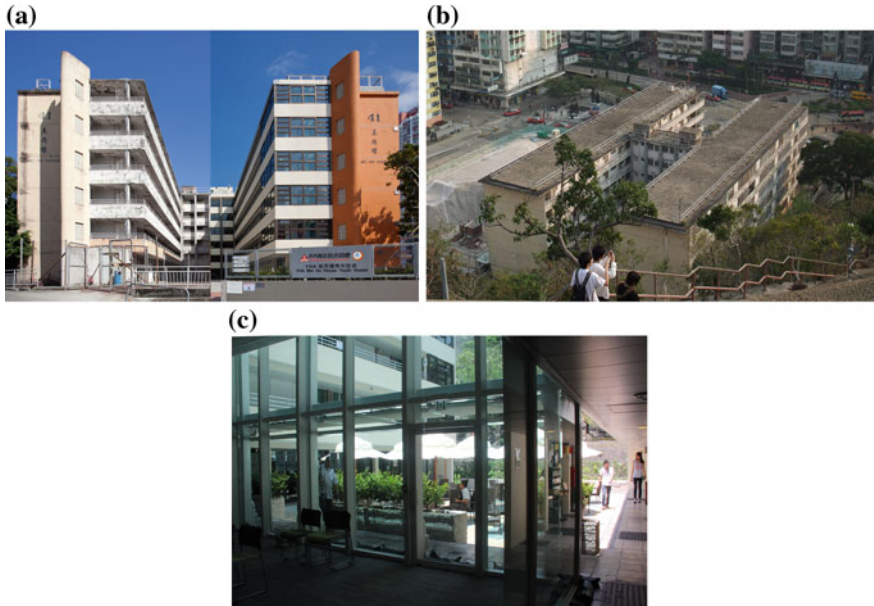
Fig. 9.9 Mei Ho Building. a Comparison of before and after renovation. Courtesy of Prof. Bernard Lim. b Before renovation, 2009. c Run as youth hostel
