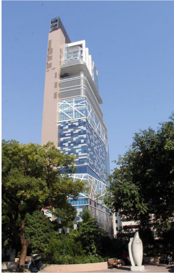
Fig. 5.15 The One, 2010. The long and narrow shape is wrapped with different pattern of curtain wall
