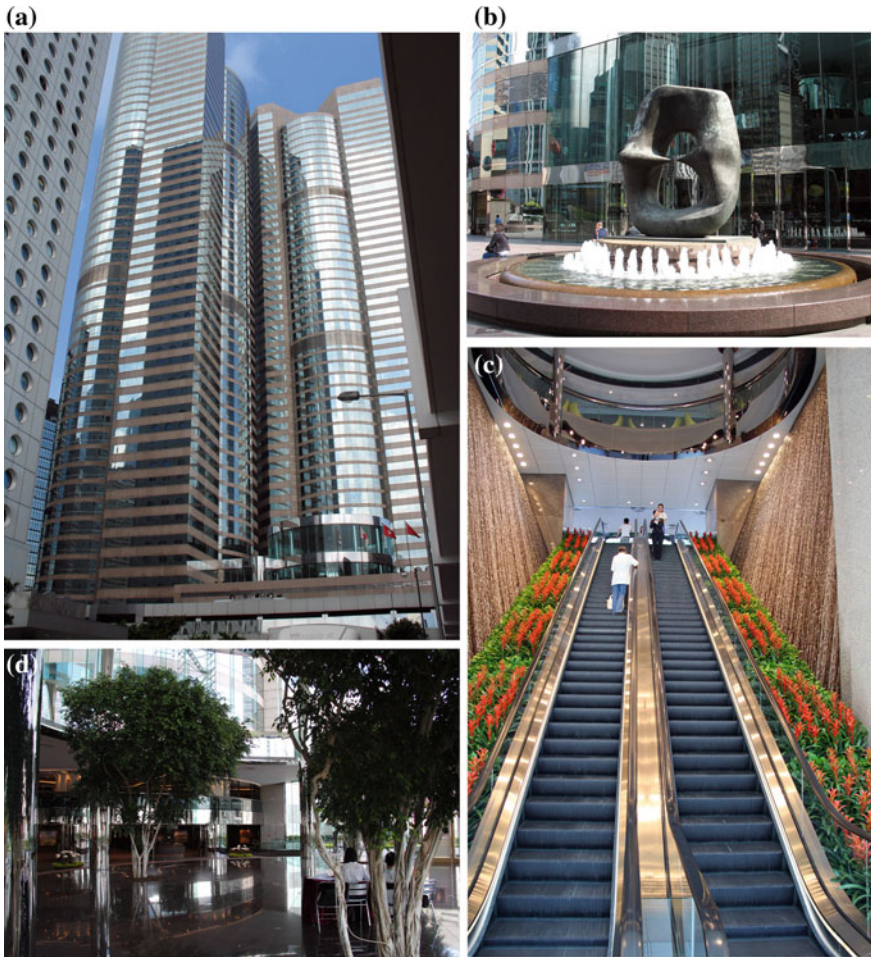
Fig. 7.15 Exchange Square, 1985. a Granite and glass form the curtain wall. b Sculpture and fountain on podium level. c From stock exchange to the office tower lobby. d Office workers and public can view the sea and occasional exhibition in the lobby
