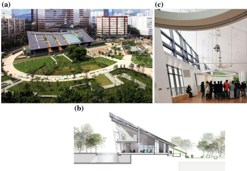
Fig. 9.14 Zero Carbon World, 2012. a Zero Carbon World is located in the old training field of CIC, now a park themed construction. b Section drawing. c Interior. Courtesy of Ronald Lu & Partners
