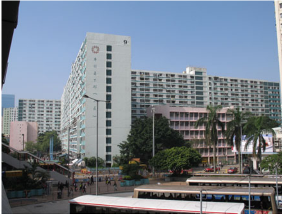
Fig. 2.9 Ngau Tau Kok Estate, 1969—the first public housing project using prefabrication. The buildings were demolished in 2009 for higher density new development
