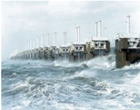
Fig. 9 The Oosterscheldekering with flood gates down during a surge event
