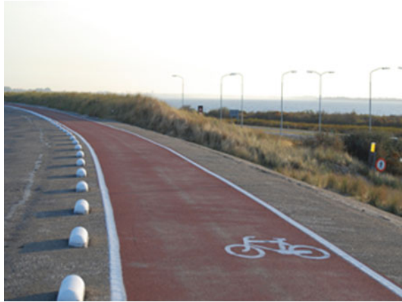
Fig. 5 View from the dam portion of Dutch coastal barrier looking inland. Reproduced by permission of William Seitz
