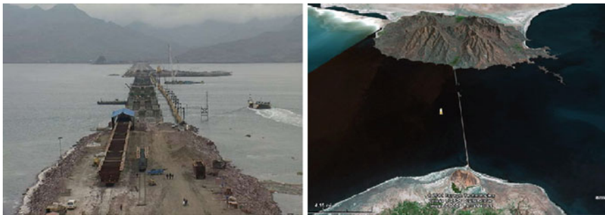
Fig. 2 Shahid Kalantari causeway across Urumia Lake; left side : construction in early stages; right side : causeway divides the lake into two separate parts (tebyan.net 2009)
