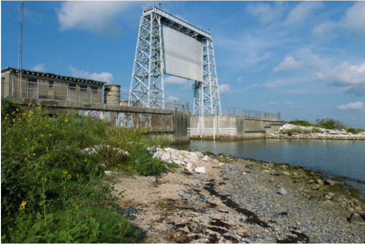
Fig. 11 The Moses Lake Flood Gate is part of an encircling flood barrier protecting Texas City and La Marque, Texas. Reproduced by permission of the Galveston County Daily News
