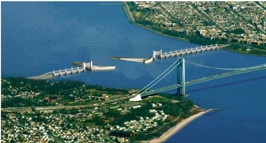
Fig. 14 Verrazano Narrows storm surge barrier design has gate combinations to assure both navigation and water circulation. Reproduced by permission of P.L.M. Jansen and P.T.M. Dircke, ARCADIS
