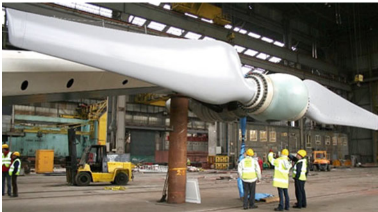
Fig. 19 SeaGen under construction
