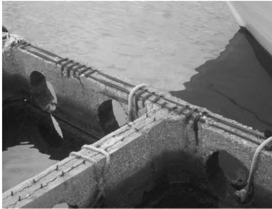
9.1 Example of chloride-induced reinforcement corrosion in concrete exposed to sea water
