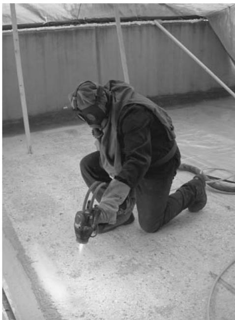
9.8 Sacrificial cathodic protection of steel in concrete by thermal zinc spraying
