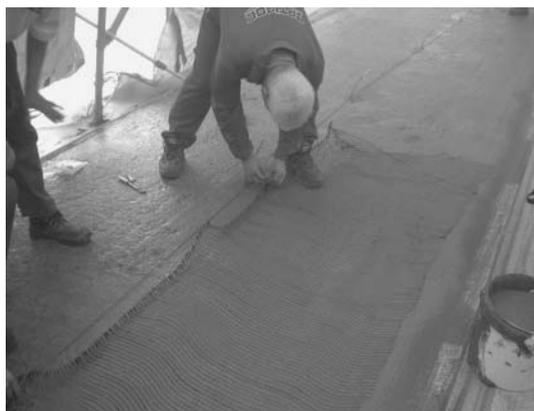
9.9 Cathodic protection by impressed current using a carbon mesh anode in a special mortar
