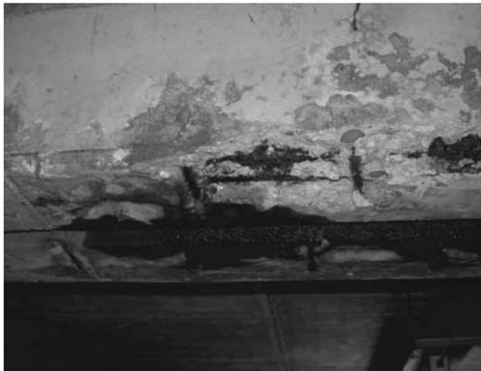
9.2 Example of chloride-induced corrosion of reinforcement exposed to de-icing salts within a leaking joint of a parking garage
