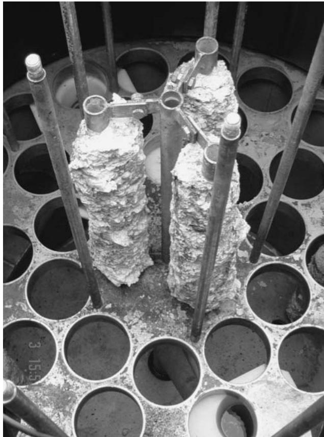
13.7 Aluminium anodes protecting the inside of a stainless steel sea water filter
