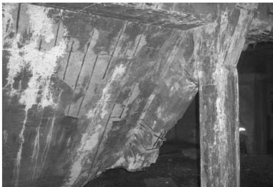
9.3 Corrosion of the reinforcement of an old concrete structure caused by insufficient concrete cover
