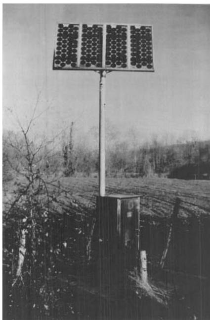
13.6 Using photovoltaic solar cells in the 1980s (France)
