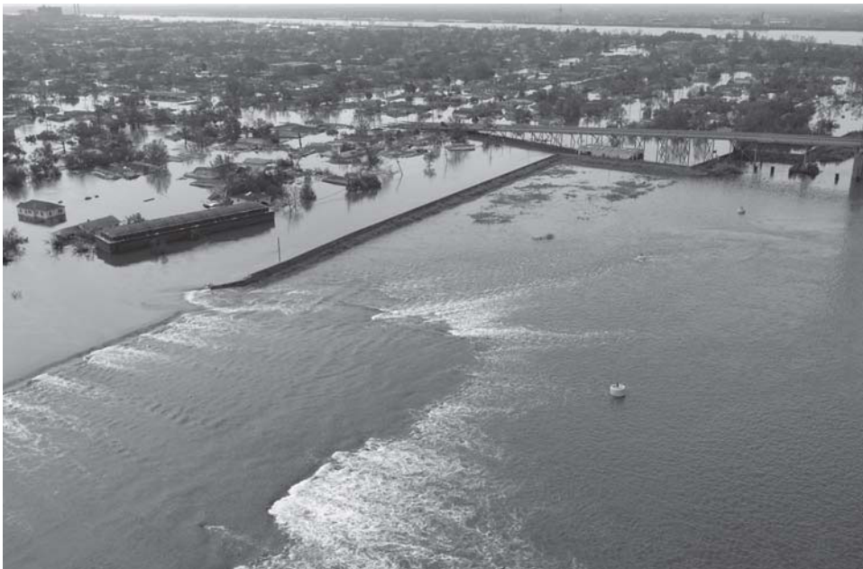
Figure 16.1 When the levees failed during Hurricane Katrina in 2005, impacts were highest in the poorest parts of New Orleans (photo: Jocelyn Augustino, FEMA).
