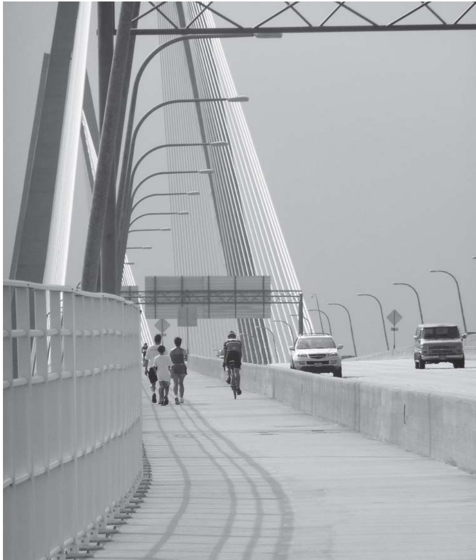
Figure 2.4 When the Arthur Ravenel Jr. Bridge crossing the Cooper River in Charleston, South Carolina, was designed (to replace an old bridge), community leaders successfully argued for adding a pedestrian and bicycle path to the span, despite the extra costs; use of the path for both recreation and transportation has far exceeded expectations (photo: Greg Yount).
