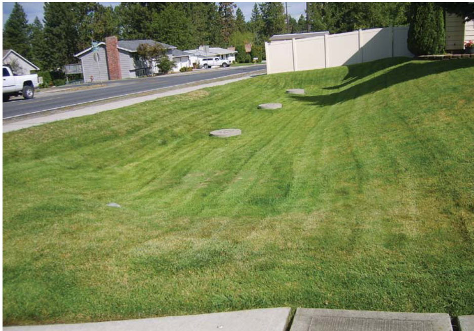
Plate 4 Swales (land depressions) are designed to help manage storm water runoff by slowing water flow and filtering pollutants and also promote rainwater harvesting and soil conservation (photo: Courtesy of City of Spokane, Washington).
