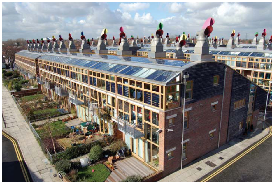
Plate 16 The design of the mixed-use Beddington Zero Energy Development (BedZED) in south London encourages sustainable, healthy lifestyles, including energy from renewable sources, efficient water and energy use, waste recycling, and travel by walking, bicycling, and public transit (photo: Tom Chance, Bioregional).
