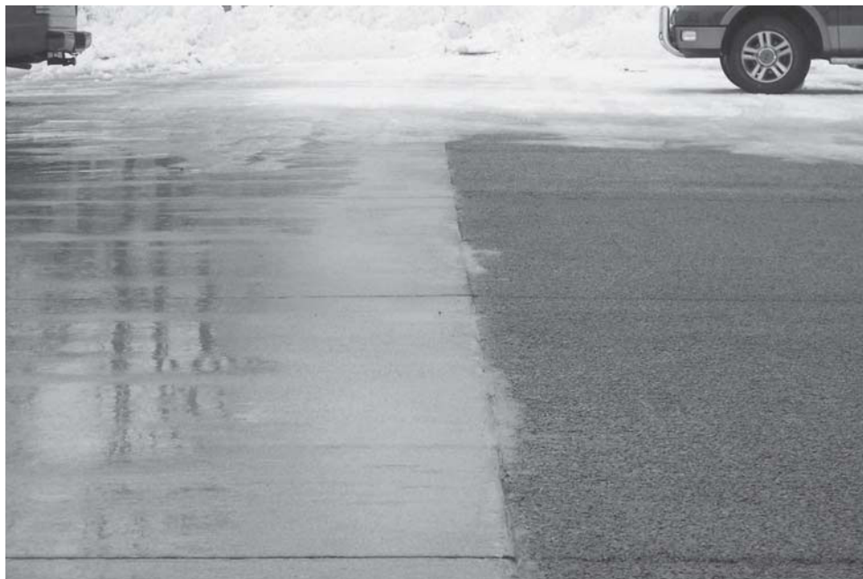
Figure 6.2 As investigated in this demonstration at Iowa State University, pervious concrete (on the right) handles stormwater runoff, urban heat island, safety, and freezing issues better than impervious types of pavement (on the left) (photo: John T. Kevern).
