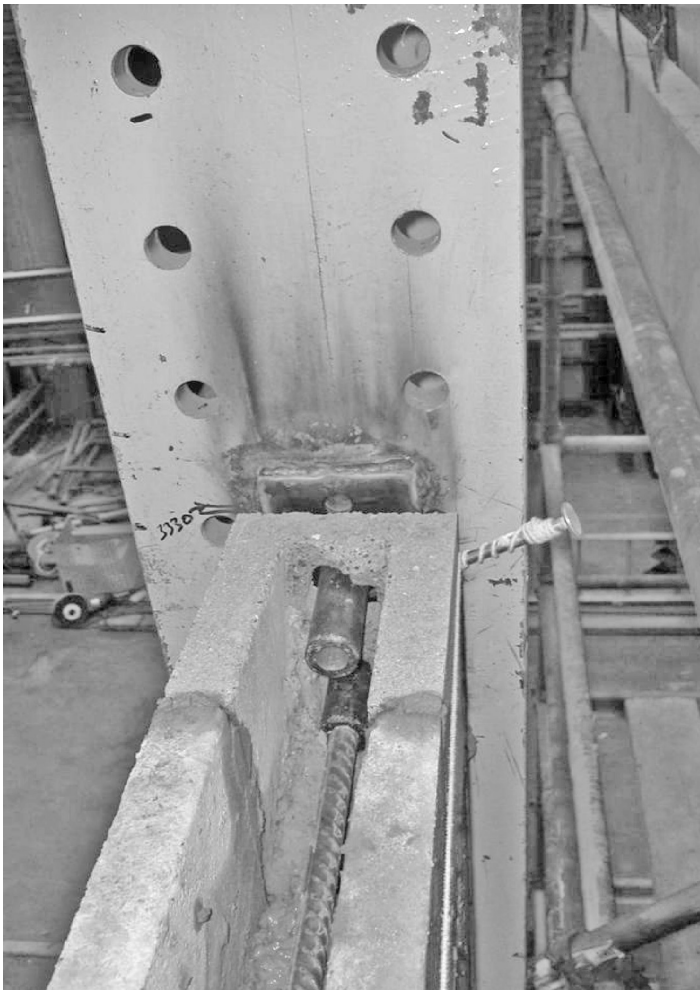
Figure 3 WI beam construction cleat detail
