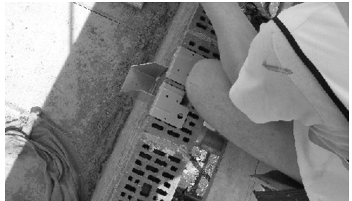
Figure 2 Traditional plus novel hangers
