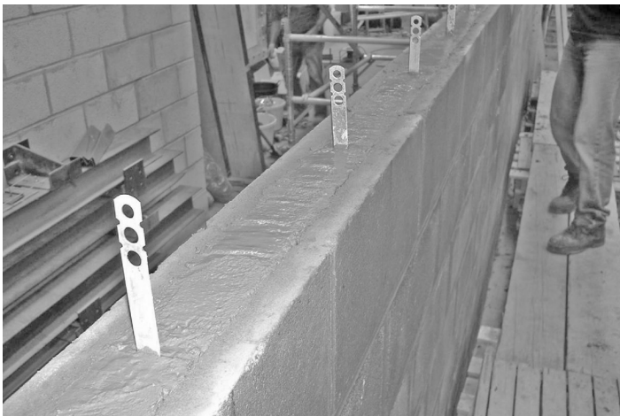
Figure 4 WI beam construction shear connectors
