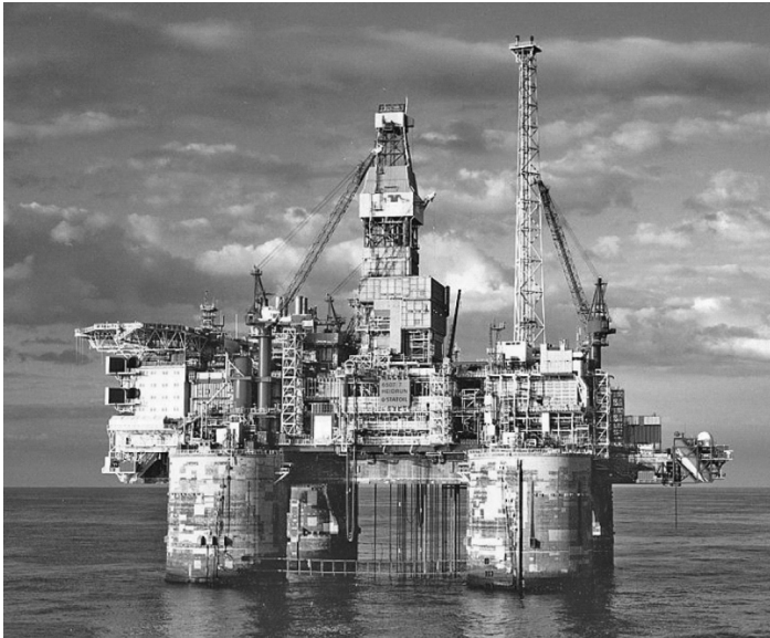
Figure 1 The Heidrun floating platform constructed out of lightweight aggregate concrete (courtesy of Elkem Materials Inc.)
