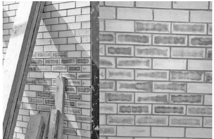
Figure 10 (a) and (b) Vanadium staining. Once seen never forgotten. Typified by vivid yellows and green staining on buff and pale cream fireclay bricks
