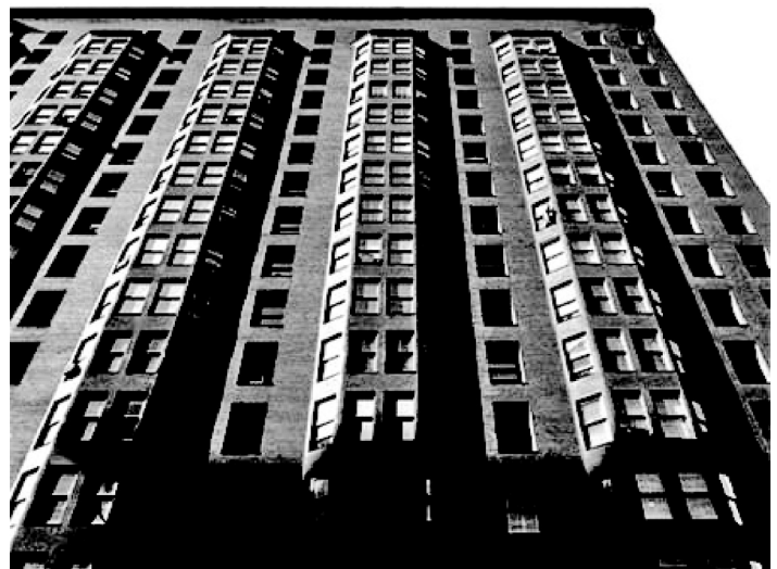
Figure 8 Monadnock Block skyscraper, Chicago, USA
