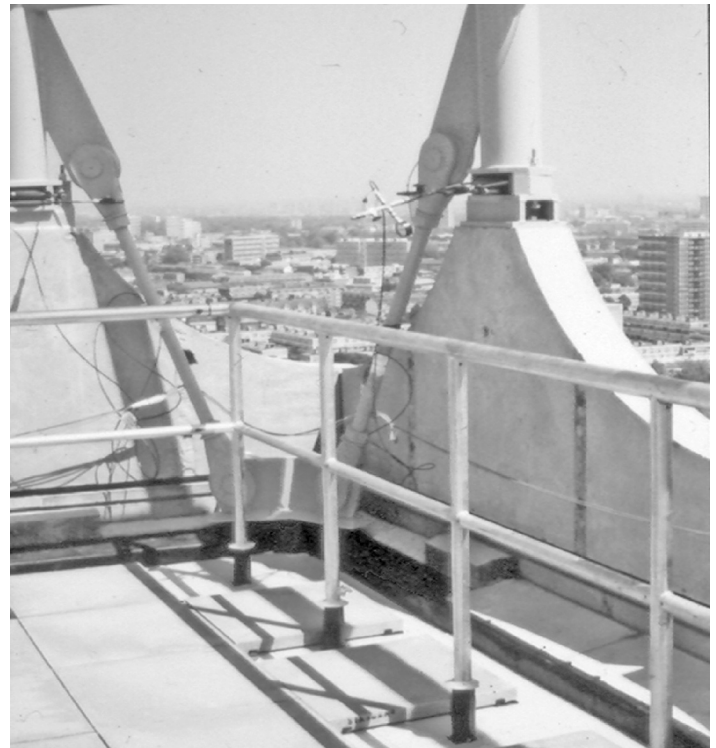
Figure 7 Winterton House support to transfer structure
