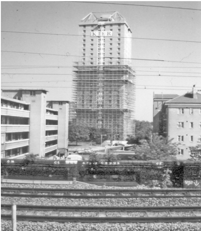
Figure 6 Winterton House general view
