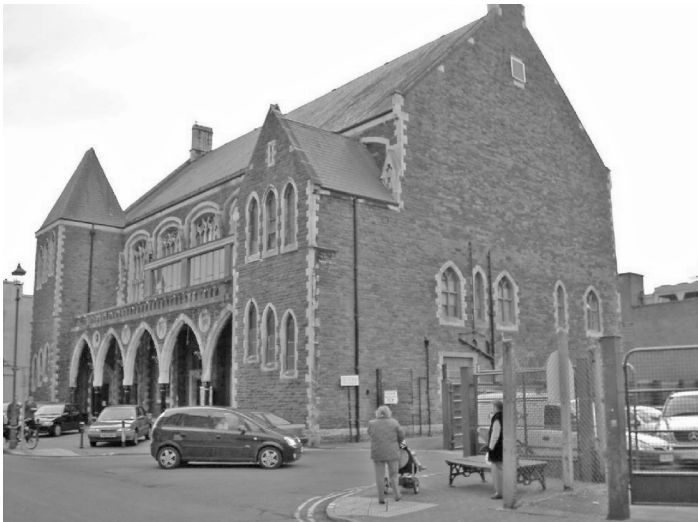
Figure 31 Gwyn Hall, Neath, South Wales
