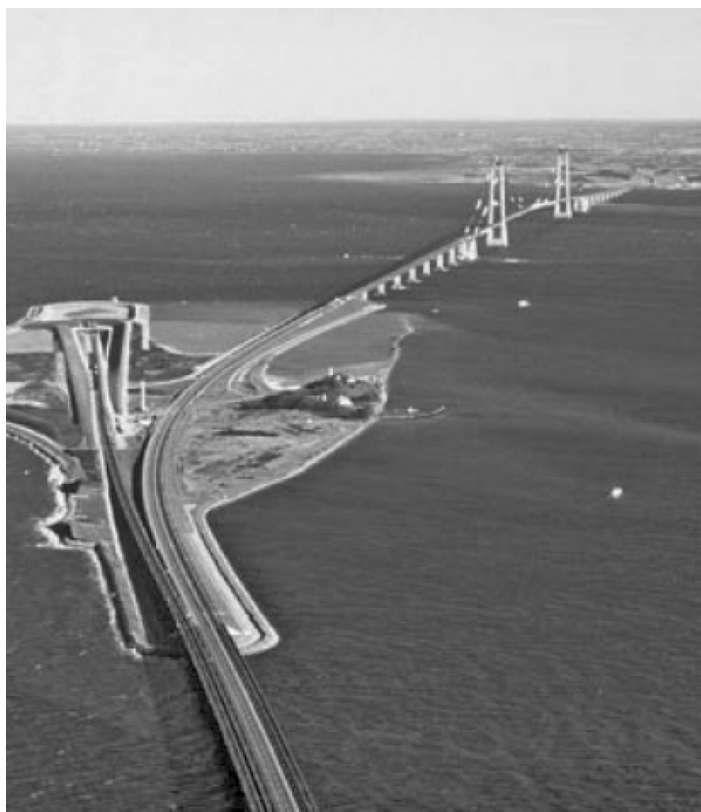
Figure 3 The East Bridge of the Great Belt Link in Denmark was designed for a life span of 100 years
