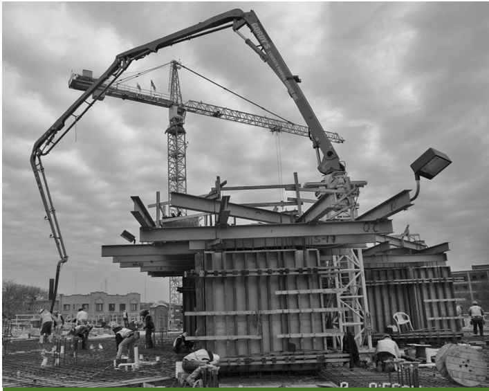
Figure 3 Pumping and placement of superplasticised concrete (Park Lafayette Tower, Milwaukee)
