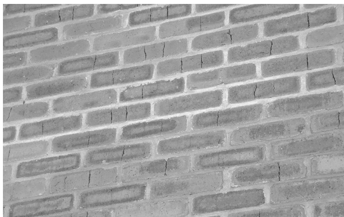
Figure 15 A wall built using fired cracked bricks
