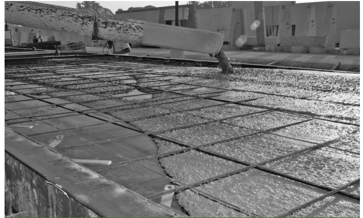
Figure 7 Self-compacting concrete used in vibrator-free precast. Note the slow creeping flow that enables full encapsulation of the reinforcing bars but without aggregate separation and blocking behind the bar. See also the self-levelling with no build-up, even at the point of discharge, and the lack of segregation so that aggregate can still be seen at the top surface with no indication of bleed water or grout separation on the leading edge
