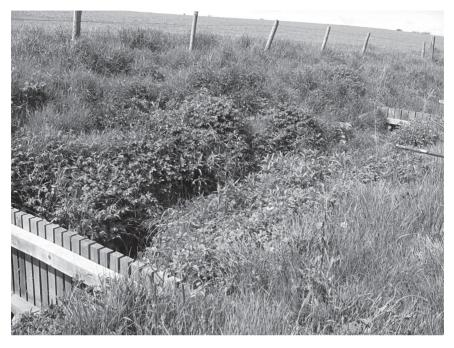
Fig. 19.10 'Leaky weirs' installed in surface water drainage ditches at Nafferton Farm to test runoff attenuation measures.
