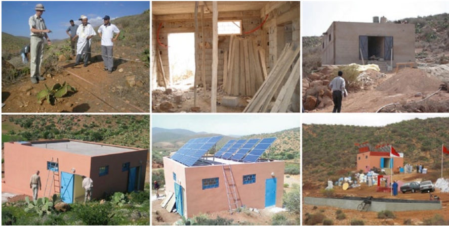
Fig. 22.8 Process of the building construction in Amellou
