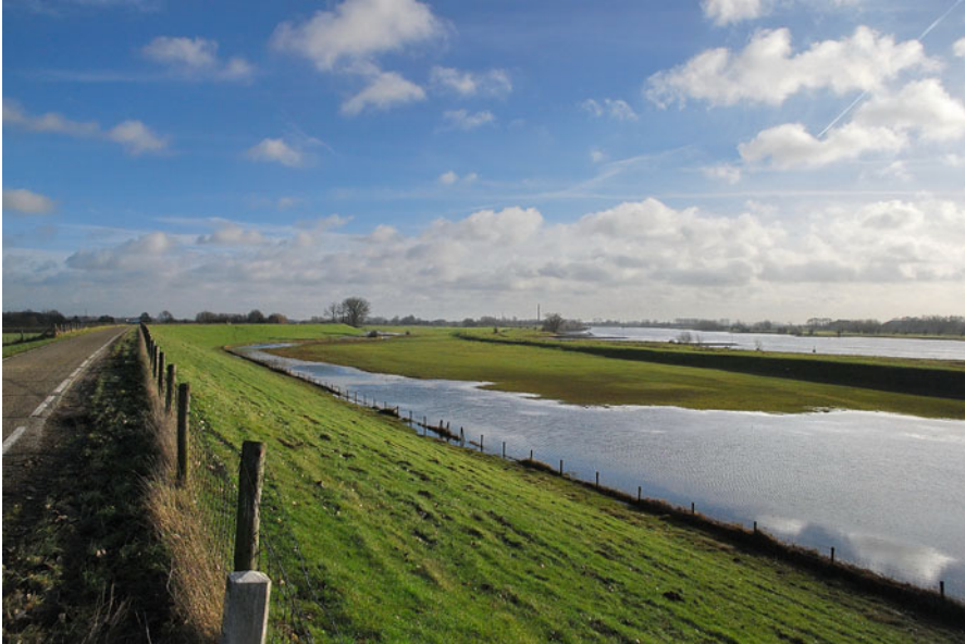
Fig. 2.1 An example of a dike structure along the river Rhine that consists of a smaller summer dike and the higher winter dike (to the left ) (Photo by W.S. van Leeuwen)
