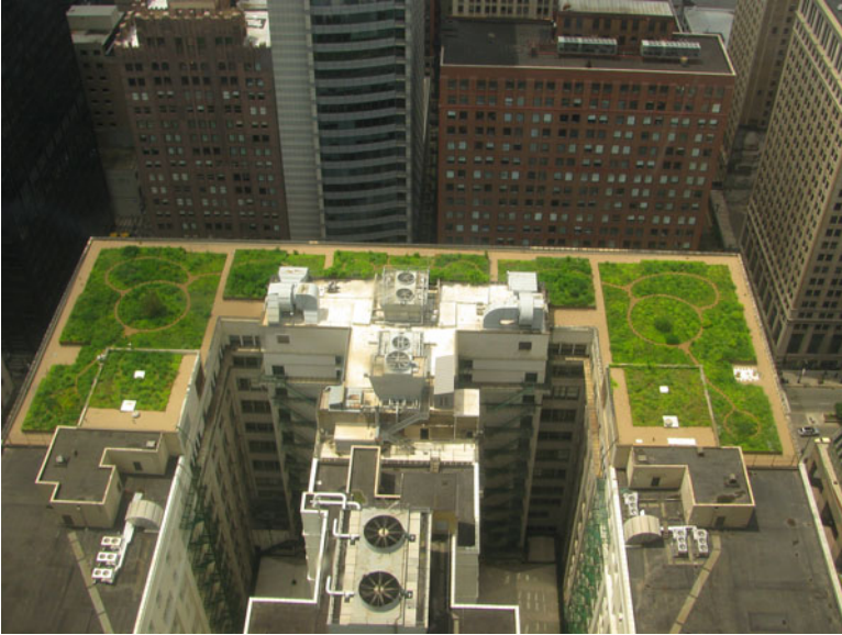
Fig. 4.4 Chicago city hall green roof (TonyTheTiger, http://commons.wikimedia.org/wiki/Main_Page )
