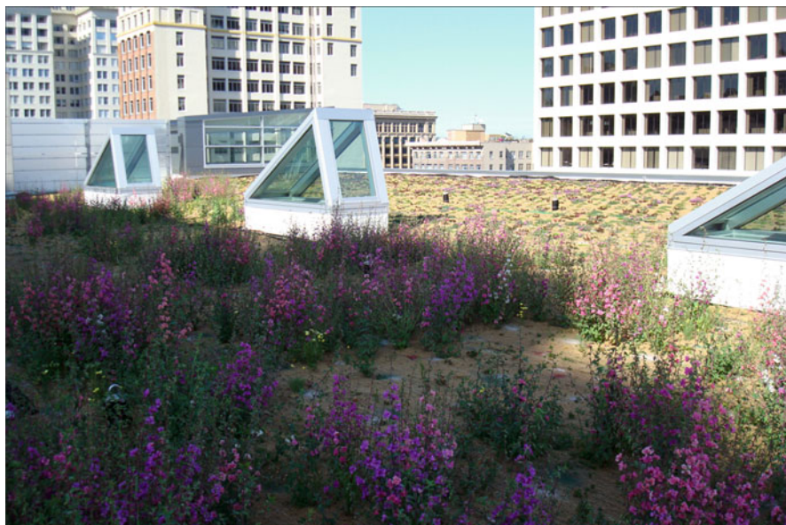
Fig. 9.2 Green roof picture. A green roof in Tacoma, WA. The soil material for this roof was made from urban organic residuals including municipal biosolids and woody debris (Photo credit: Dan Thompson)
