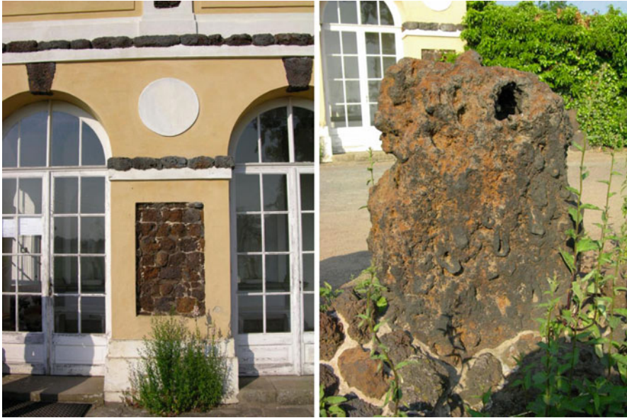
Fig. 1 Left: Bog iron used as building material for a house, Wörlitzer Park, Germany. Right: Exhibit of a large specimen of bog iron, Wörlitzer Park, Germany
