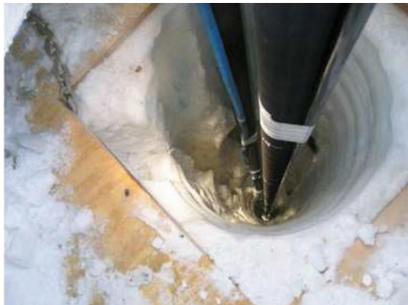
Fig. 10.12 The hot water hose and support cables disappear down one of the many boreholes drilled into the Antarctic ice to construct the IceCube Neutrino Observatory. Credit: Jim Haugen, IceCube/NSF
