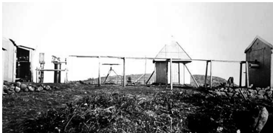
Fig. 5.8 The American transit of Venus station at Nagasaki. Features from left to right are: the 'transit house'; the weight drive and adjacent pier holding the heliostat; the wooden framework leading towards the photographic house; the 'equatorial house'; and part of the 'photographic house' (courtesy: transitofvenus.nl/wp/past-transits/1874-december-9/ )
