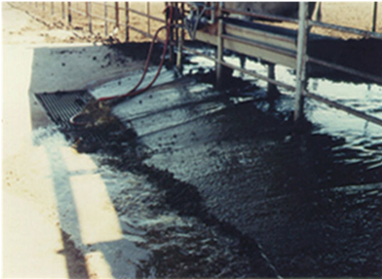
Fig. 5.18 Receiving pit for flush dairy dry lot (Photo courtesy: AgSTAR)
