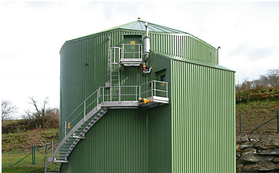
Fig. 7.10 A BIMA digester processing 11,000 tonnes per year of municipal sewage sludge at Tamsweg, Austria (photo courtesy: Entec biogas)
