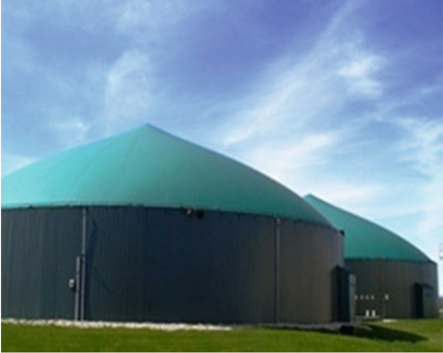
Fig. 5.14 Completely mixed digester (Photo courtesy: AgSTAR)
