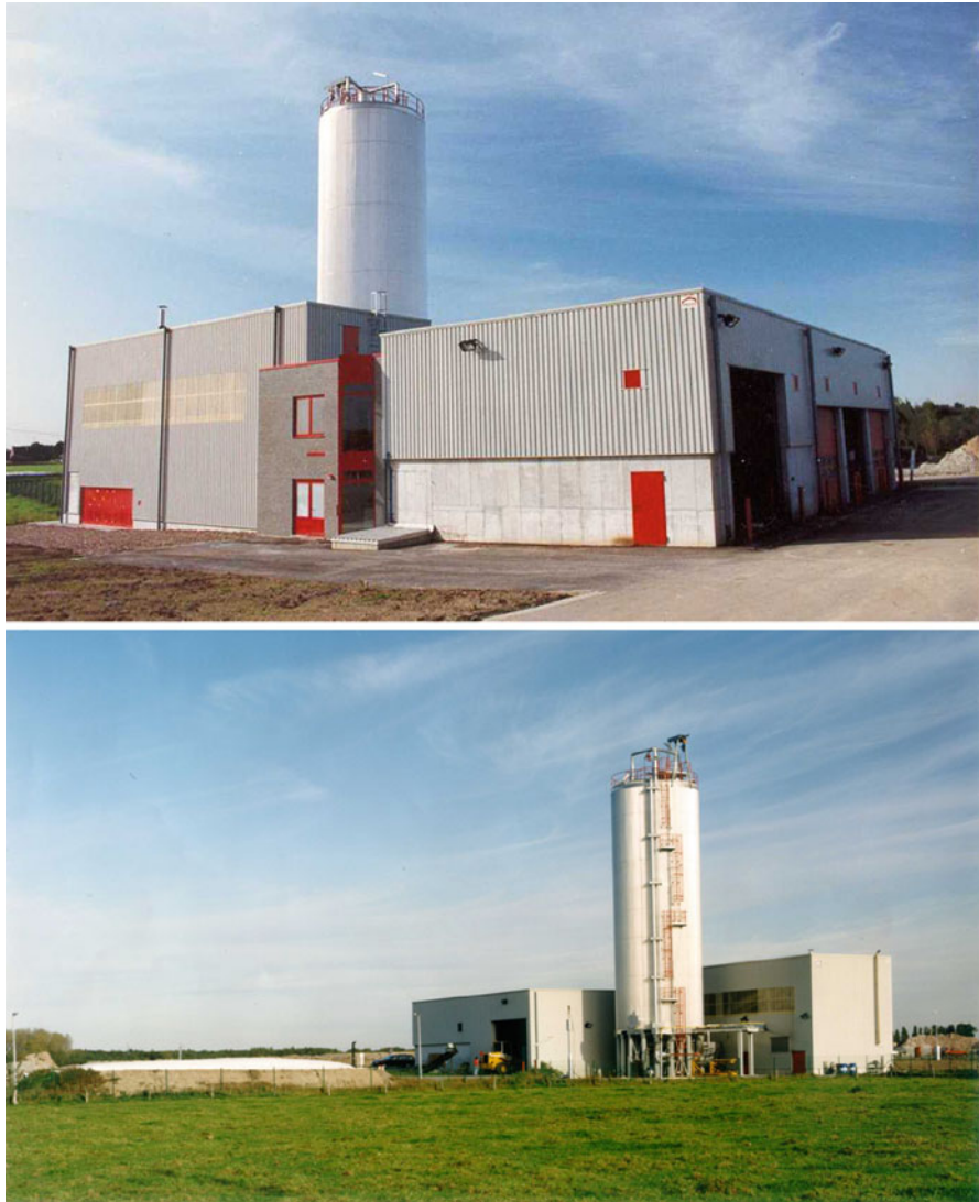
Fig. 7.24 Front ( top ) and back views of the DRANCO plant at Brecht (Belgium) treating non-recyclable wastepaper, cardboard, disposable diapers, etc., at 70,000 tonnes per year capacity since 1992 (photo courtesy: Organic waste systems n.v.)
