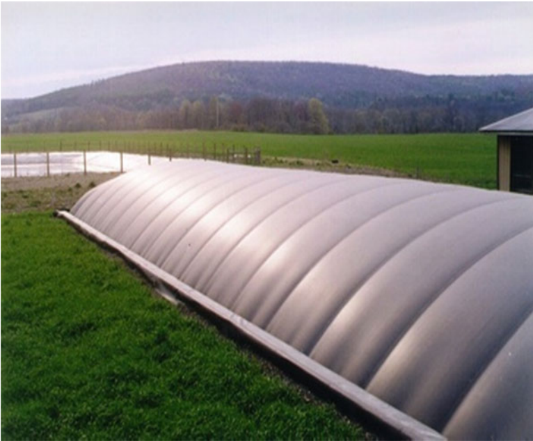
Fig. 5.11 Plug-flow digester (Photo courtesy: AgSTAR)
