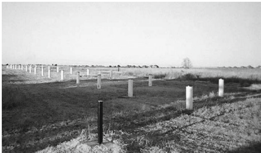
Fig. 11.3 Photo of a 215 m proton reduction system currently operating at an Oklahoma site (USA). The system functions as a permeable reactive barrier to eliminate off-site migration of chlorinated solvents, and it has been in operation successfully for >3 year
