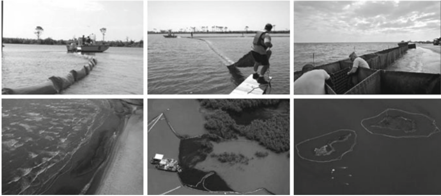
Fig. 24 Protection works around shores and islands (DWHR)
