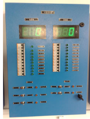
Fig. 3. The DC power distribution box
