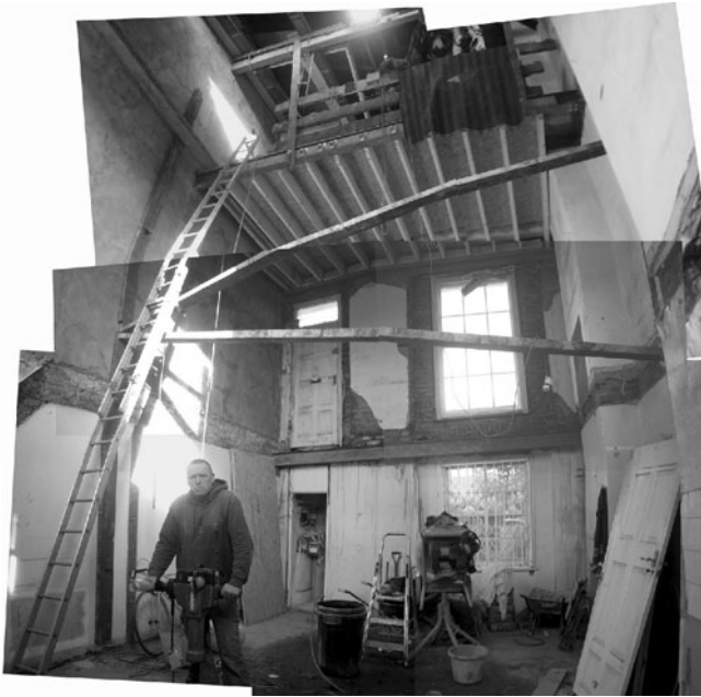
Figure 5.2 'Site Progress', Victorian conversion, Hackney, 2009
