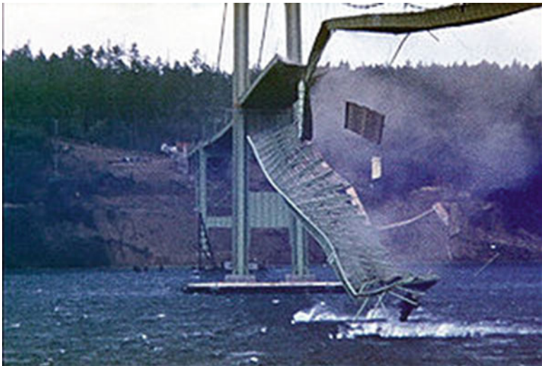
Fig. 18.1 The Tacoma Narrows Bridge collapse on November 7, 1940 (Photo taken by Barney Elliott, presented according to fair-use principles)
