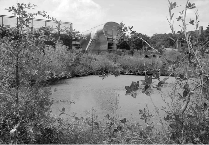
Figure 5.2 Many cities have begun to turn underused sites into water-retaining landscapes that also add value to neighborhoods, like this water-treatment plant in Hamden, Connecticut, where the planted roof blends seamlessly into the landscape (Steven Holl, architect, and Michael Van Valkenburgh, landscape architect). Credit: James S. Russell
