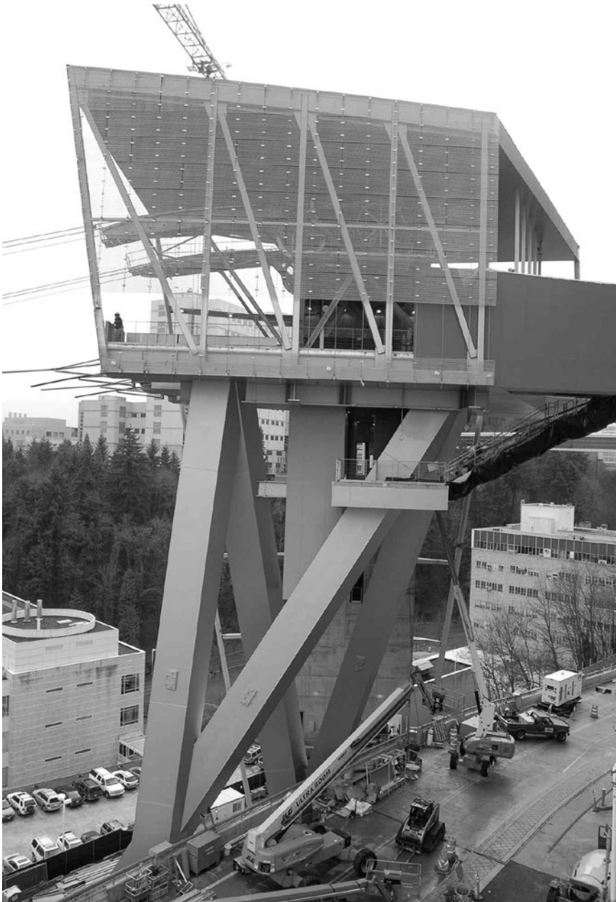
Figure 9.1 A stylish aerial tram links the hilltop Oregon Health and Science University and expanded facilities in the South Waterfront mixed-use development, in Portland. Credit: James S. Russell
