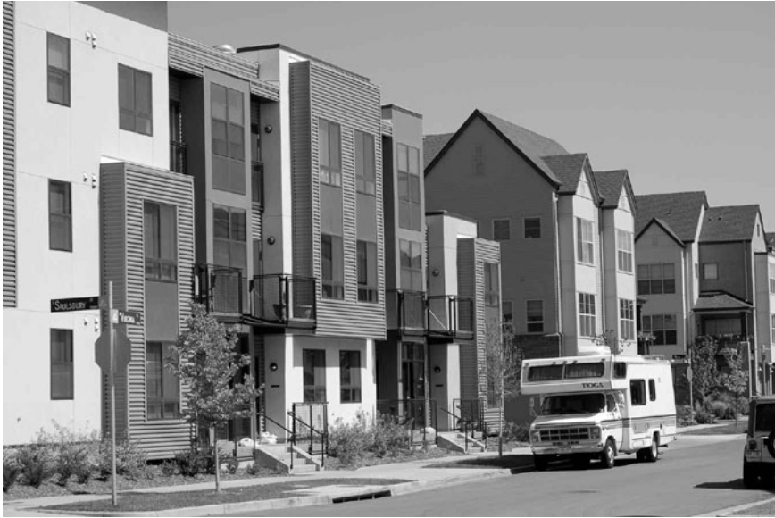
Figure 9.2 The Belmar development, outside Denver, replaced an obsolete shopping center surrounded by parking with a mixed-use community that includes lofts, artists studios, and an art museum ranged along a network of streets and squares. Credit: James S. Russell
