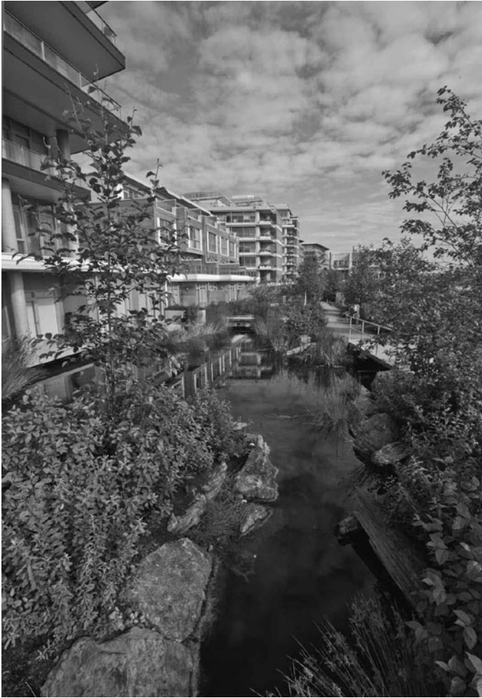
Figure P.4 At Dockside Green, storm runoff and water treated in an on-site sewage plant combine in a naturalized stream that creates an amenity for residents as it keeps polluted water out of Victoria's sparkling Inner Harbor. Credit: Courtesy Dockside Green
