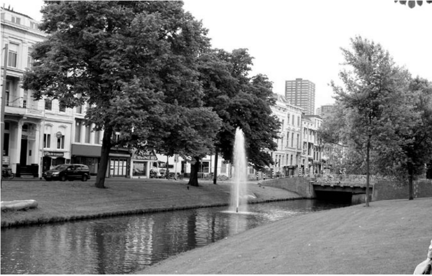
Figure 5.4 The Westersingel Canal, in Rotterdam, is configured to retain excess water during storms and to release it when the water system is no longer overloaded. Credit: James S. Russell
