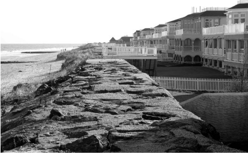
Figure 2.2 High walls have long protected the beach town of Sea Bright, New Jersey, because development too close to the shore prevented the beach from replenishing itself. Repeated replenishment with offshore-dredged sand prevents the beach from narrowing. Credit: James S. Russell
