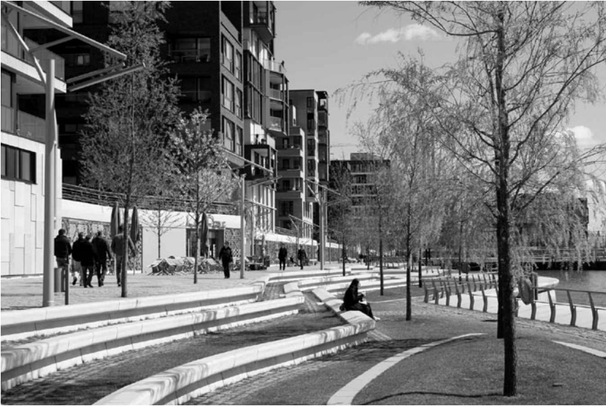
Figure 8.6 While buildings at HafenCity, in Hamburg, are raised above flood levels, a lower-level esplanade is resilient to floods. Heavy doors slide into place in the event of high water to protect cafés that line the walkway. Credit: James S. Russell
