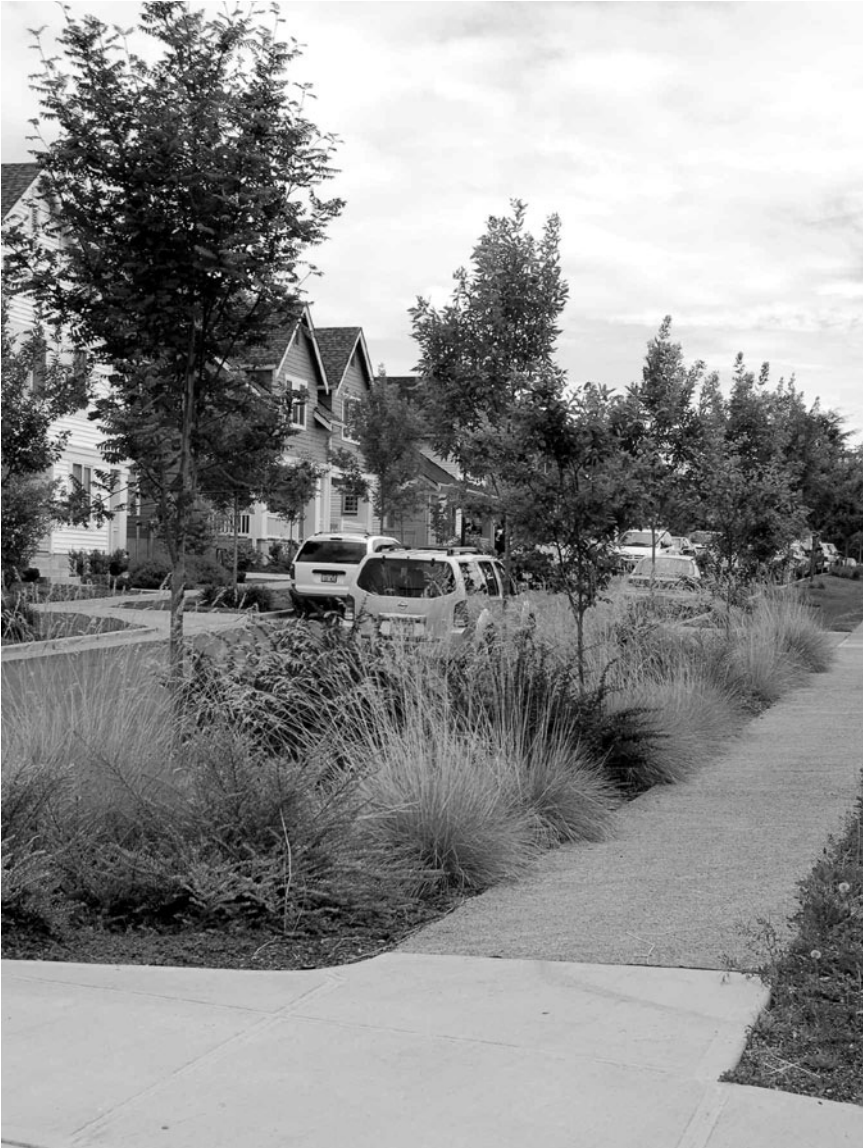
Figure 9.5 Although storm water–absorbing rain gardens, like this one in the High Point redevelopment in Seattle (Mithun, architects), are rapidly becoming popular, they must still be made legal in many localities. Credit: James S. Russell
