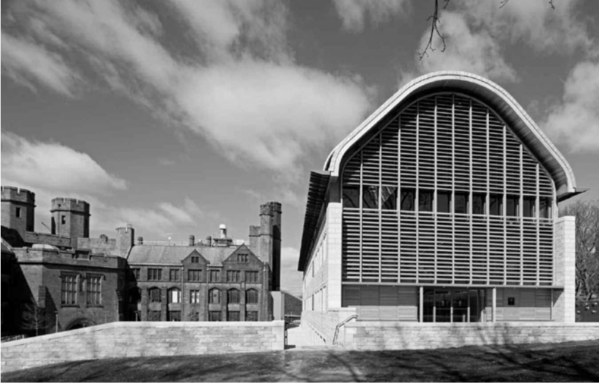
Figure P.1 Kroon Hall, Yale University. The louvers on the east-facing side of this building are one of many tactics designed by Hopkins Architects with Centerbrook Architects to achieve near zero-carbon emissions. Credit: © Robert Benson
