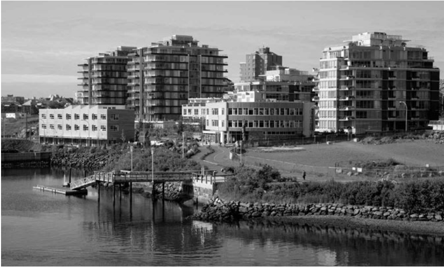
Figure P.3 Overview of the early phases of Docksider Green, in Victoria, British Columbia. Its location near downtown allows residents to get to destinations along a bike path that runs along the Inner Harbor and on a passenger ferry that crosses it. Credit: Courtesy Docksider Green
