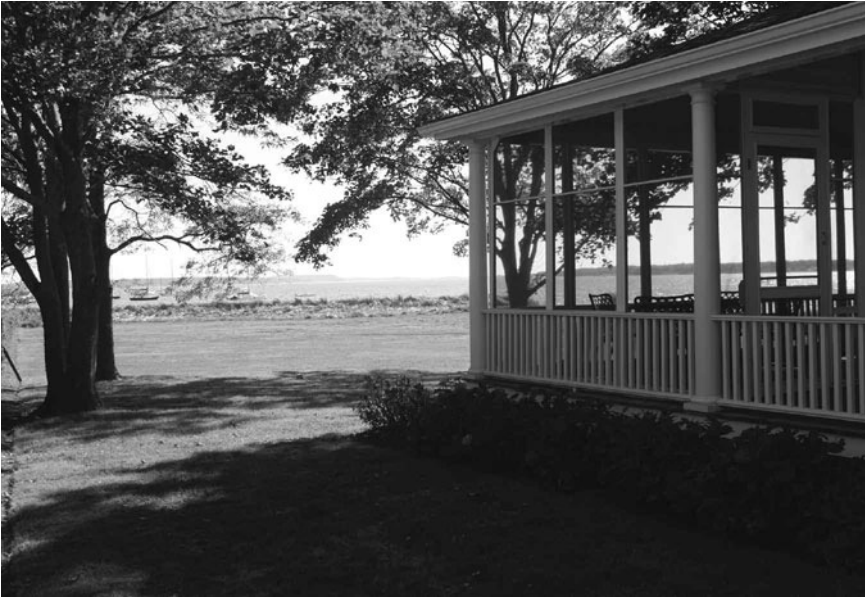
Figure 7.1 Along the northeastern seaboard, climate-sensitive houses orient porches to capture summer breezes and funnel them through the cross-ventilated houses. Credit: James S. Russell
