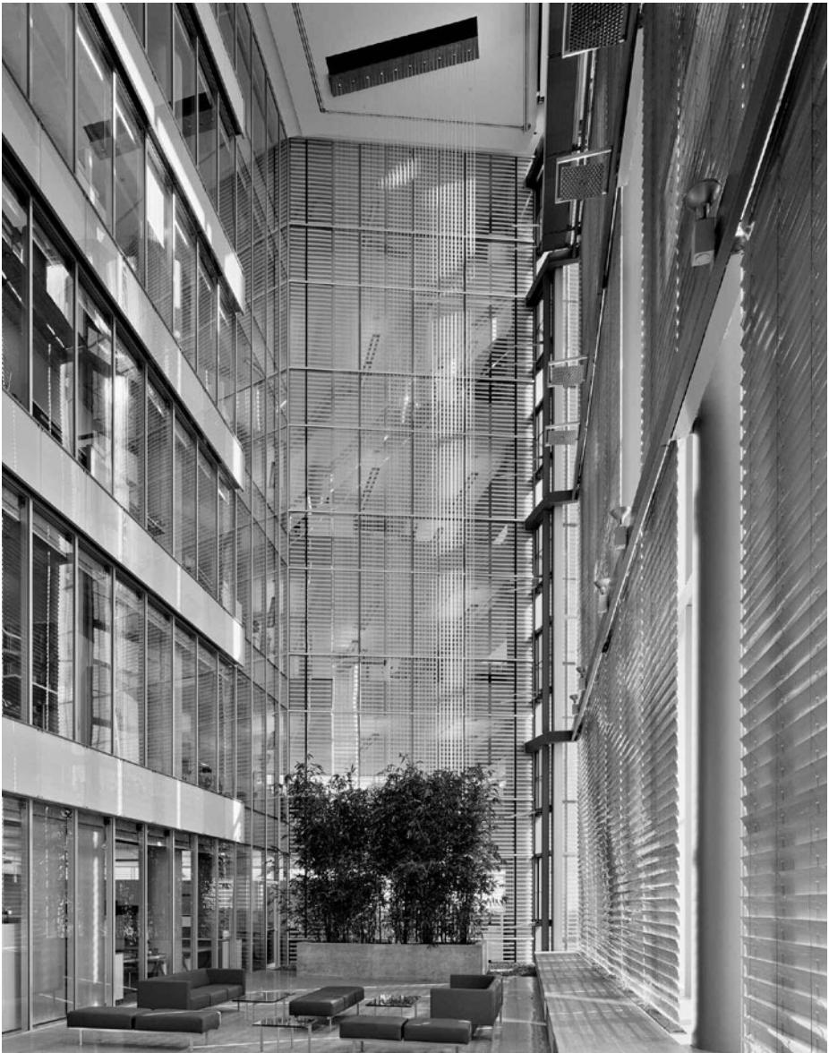
Figure 7.5 The tall winter gardens in the Manitoba Hydro building act as a thermal blanket in winter, “preheating” the building with a combination of strong winter sun, heat recycled from air exchangers, and heat generated from a geothermal well system. Credit: © Eduard Hueber, courtesy KPMB Architects
