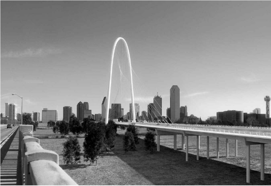
Figure 8.1 A bridge designed by Santiago Calatrava is one feature of the Trinity River project, in Dallas, which mixes environmental restoration and new parklands with extravagant highways and upgraded levees. Credit: Courtesy Trinity River Project
