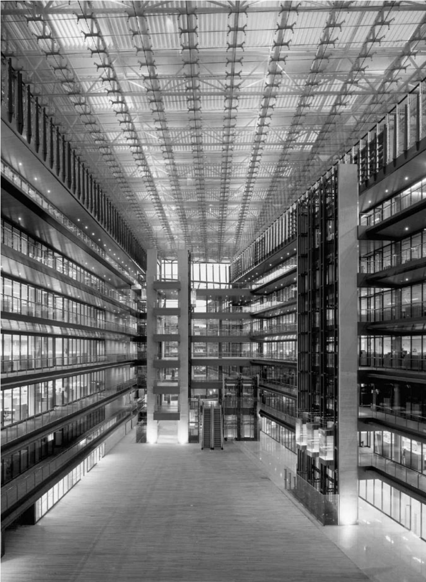
Figure 7.4 The glass roof of the Endesa headquarters outside Madrid both shades an internal courtyard and supplies daylight to offices that wrap its perimeter. Solar chimneys temper the space by exhausting warm air (KPF and Rafael de La-Hoz, architects). Credit: © H. G. Esch courtesy KPF
