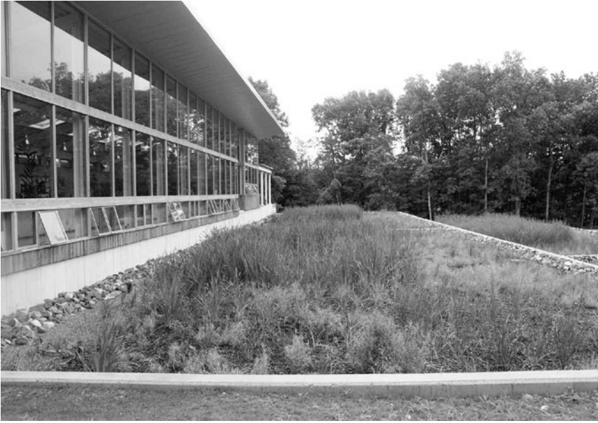
Figure 5.1 At the Center for Sustainable Living at the Omega Institute for Holistic Studies, natural wetlands “polish” sewage that has already been treated by an “Eco Machine” using plants and naturally occurring organisms. Credit: James S. Russell
