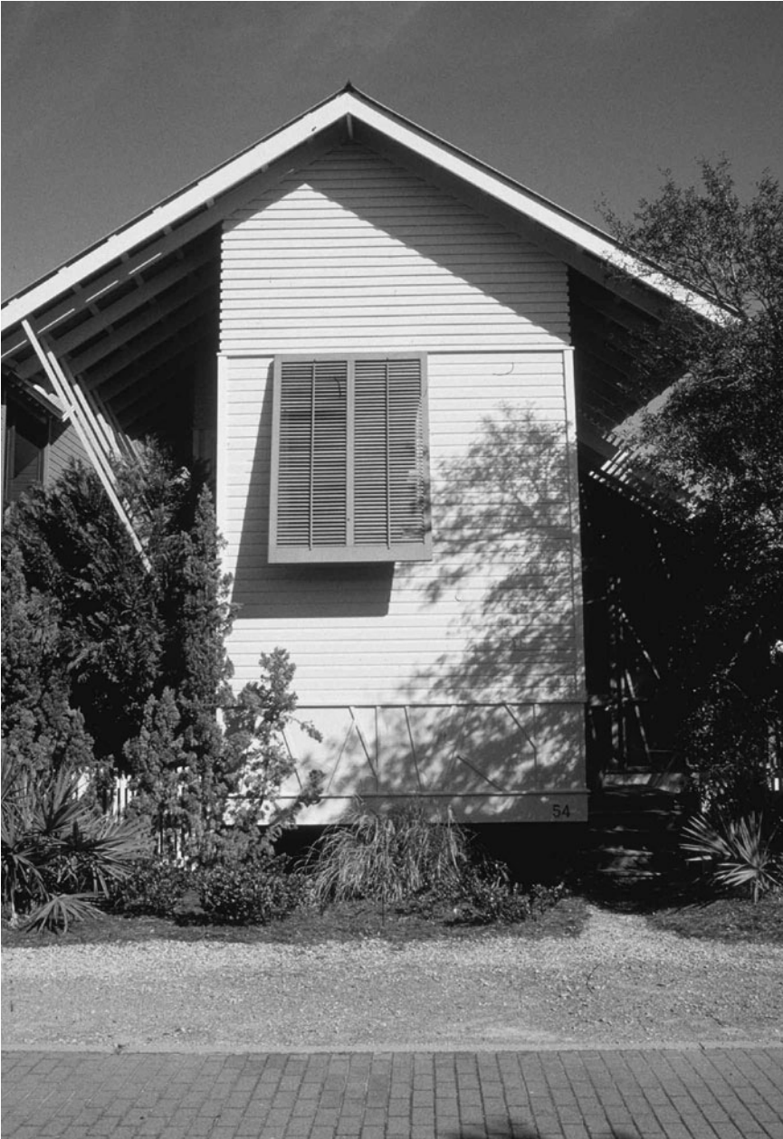
Figure 7.2 Louvered shutters cut the heat of the sun while admitting breezes and maintaining privacy. Sturdy ones can protect windows from hurricanes and intruders. Credit: James S. Russell
