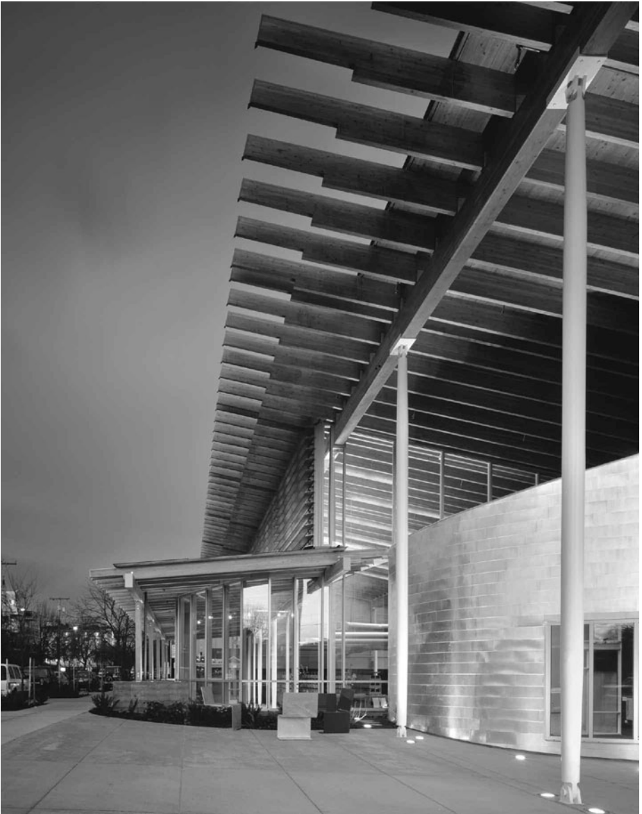
Figure 7.6 The planted roof of the Ballard Library in Seattle absorbs rain runoff and curves up to admit daylight to the reading room. Its wide roofs shelter patrons from the city's perpetual drizzle. Credit: Nic Lehoux Courtesy Bohlin Cywinski Jackson architects
