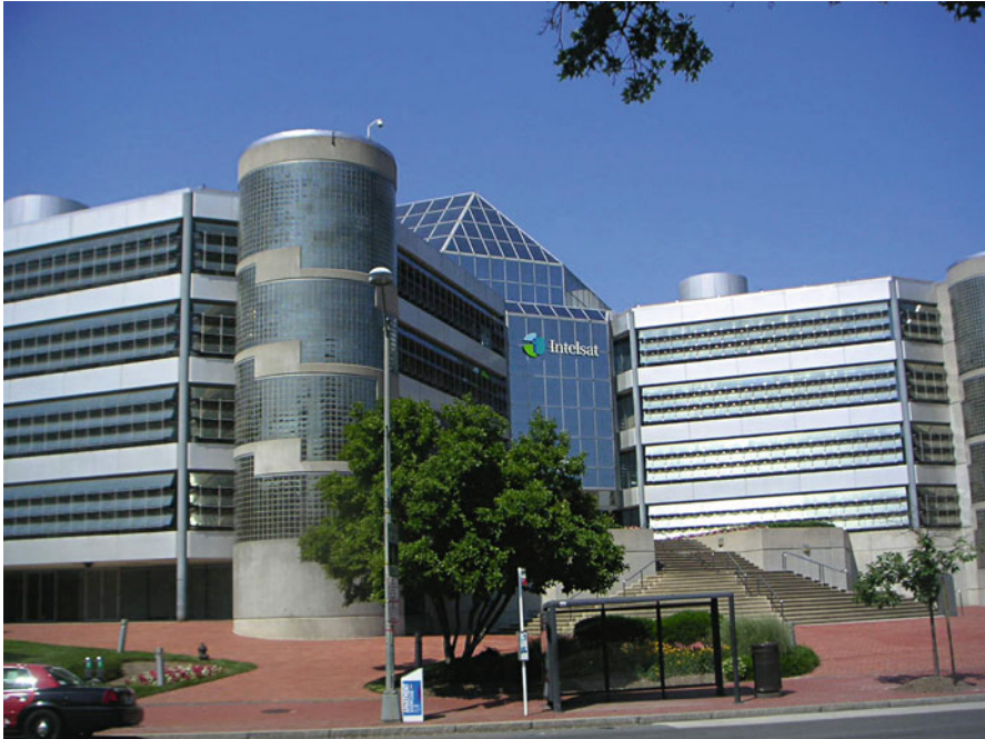
Fig. 3 The INTELSAT building in Washington, DC (Photo courtesy of Intelsat)
