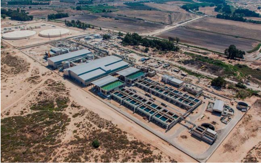
Figure 5.25 World's largest desalination plant (Sorek) 15 km south of Tel Aviv, Israel using RO technology [38]. From IDE Technologies.
