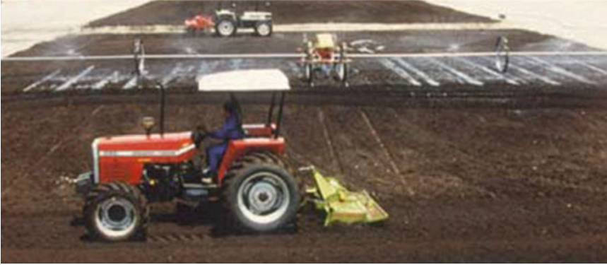
Fig. 1 Typical landfarming treatment unit
