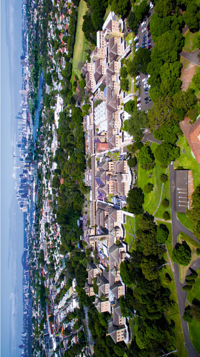
Fig. 13.1 Callan Park showing the Kirkbride Complex and proximity to Sydney, the Harbour Bridge and tip of the Opera House, February 2016 (Photographer: Jason Burcher; Retoucher: Thomas Ulman)
