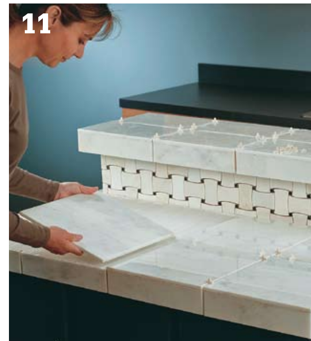
11 Install the field tiles for the countertops last (see How to Build a Tile Countertop, pages 113 to 119).
