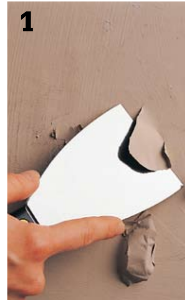
1 Scrape away loose paint with a putty knife or paint scraper.
