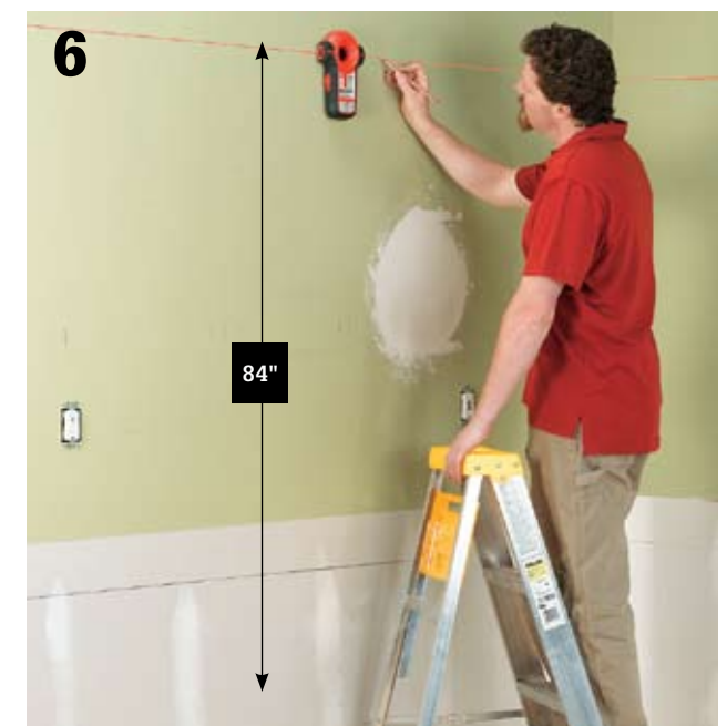
6 Measure up 84" from the high-point mark and draw a second reference line. Wall cabinets will be installed with their top edges flush against this line.
