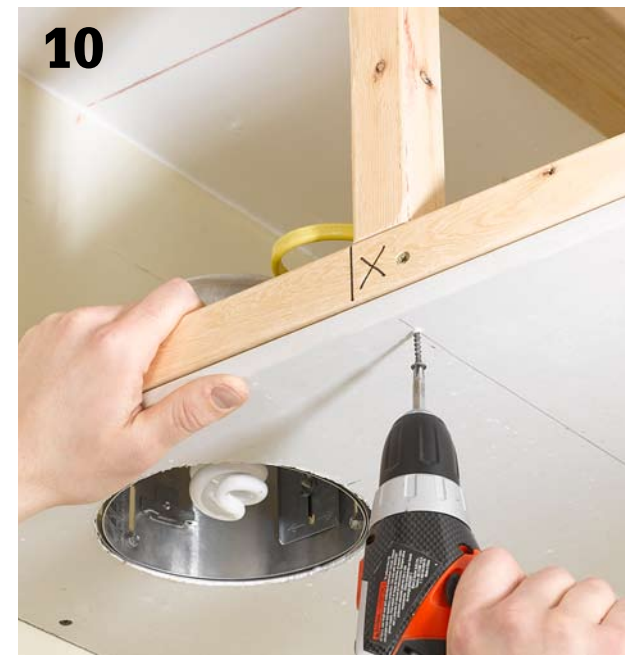
10 Cut and install 5/8" wallboard over the framework using wallboard screws. Attach the bottom sections first, then cut and attach the sides. Note: Required minimum wallboard thickness is dictated by local building codes. Be sure to consult them before you begin installing wall coverings.
