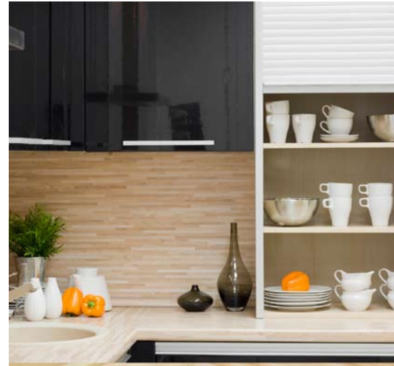
Modern results can come from the most ancient materials. This ultra-contemporary backsplash is fashioned with edge-glued strips of bamboo—just about the oldest building material known to man.
