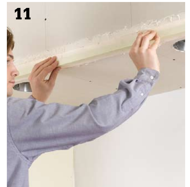
11 Apply joint compound and tape to the wallboard. Use corner tape along all the edges. Sand smooth and finish with primer and paint.
