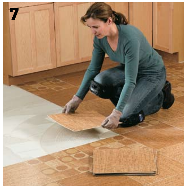
7 Complete the first three quadrants , and then spread adhesive over the remaining quadrant and finish setting the tile.
