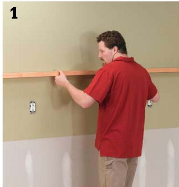
1 Find high and low spots on wall surfaces using a long, straight 2 × 4. Sand down any high spots.
