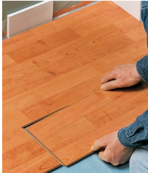
Laminate flooring comes in narrow panels or strips that have click-together tongue-and-grooved edges and ends.
