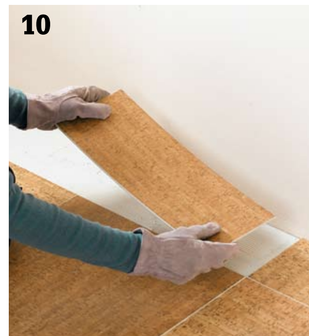
10 Install the cut tiles next to the walls. If you're precutting all the tiles before installing them, measure the distance between the wall and install the tiles at various points in case the distance changes.
