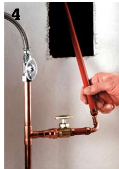
4 Attach the new PEX supply line to the T-fitting at the supply riser, installing an accessible shutoff valve on the new line.
