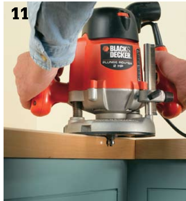
11 Pull the countertop section away from the wall a few inches, and make a roundover cut along the front edges with a piloted roundover bit.
