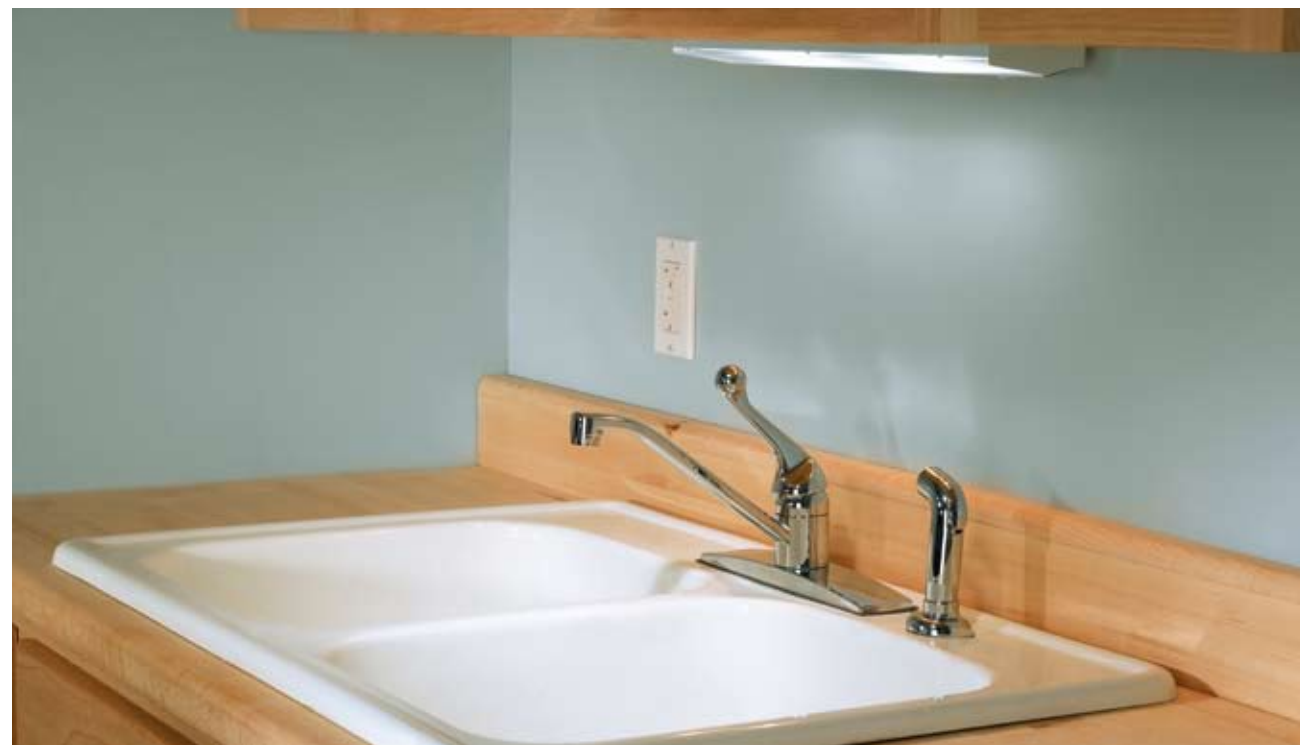
Undercabinet lights provide directed task lighting that brings sinks and countertop work surfaces out from the shadows. Hardwired lights may be controlled either by a wall switch or an onboard on/off switch located on the fixture. Note: Do not supply power for lights from a small-appliance circuit.
