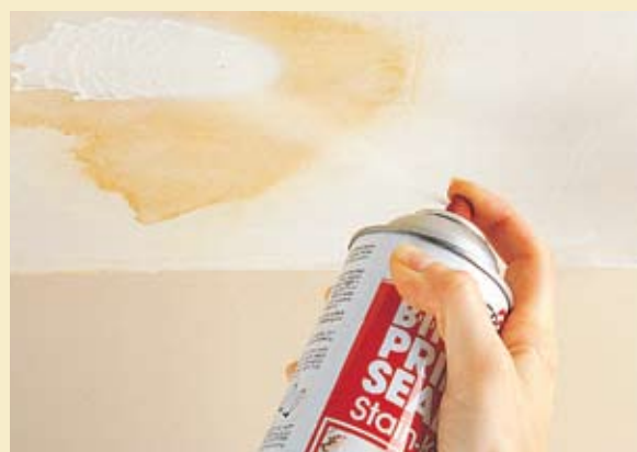
Water or rust stains may indicate water damage. Check for leaking pipes and soft plaster, make needed repairs, then seal the area with stain-covering sealer.
