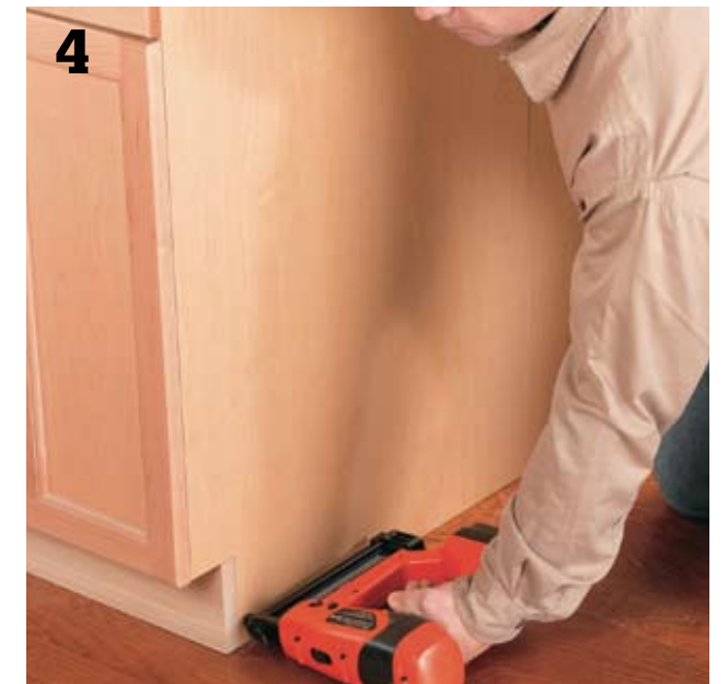
4 Attach the cabinets to the floor cleats using 6d finish nails. Drill pilot holes for nails, and recess the nail heads with a nail set. Make a countertop (see pages 86 to 123) and install it on top of the cabinets.
