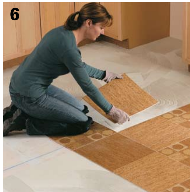
6 Spread adhesive over most of the installation area, covering three quadrants. Allow the adhesive to set according to the manufacturer's instructions, then begin to install the tile at the intersection of the layout lines. You can kneel on installed tiles to lay additional tiles.
