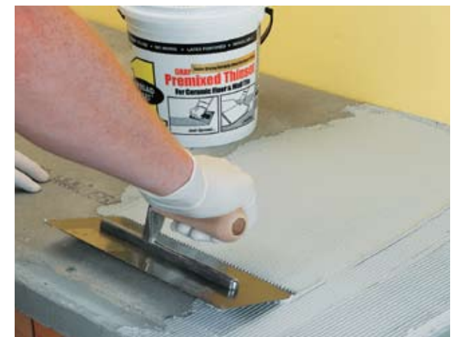
Tiles are set into a bed of thinset mortar troweled onto a cementboard or tilebacker subbase.
