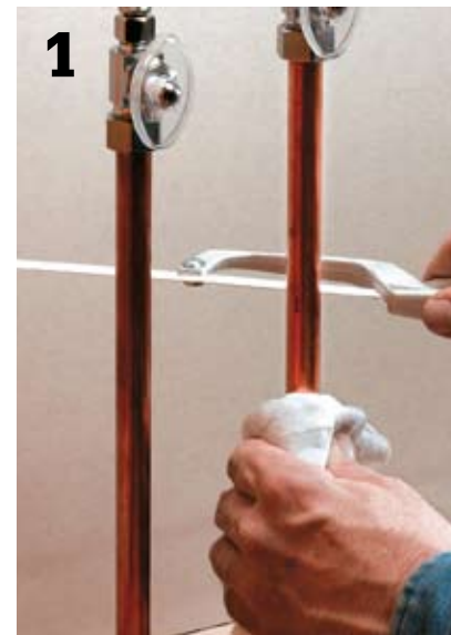
1 Shut off the water supply and locate the cold-water supply riser at the kitchen sink. Cut into the riser and install a T-fitting, or replace the existing shutoff valve on the riser with a multiple-outlet shutoff valve, with an outlet for the \frac{1}{2} " supply pipe for the pot filler.
