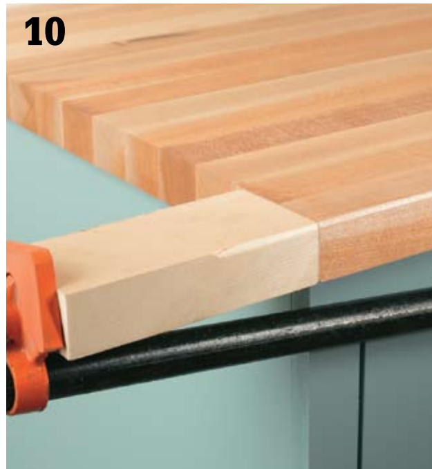
10 Clamp a piece of scrap wood to the end of the countertop so the tops are flush. The scrap wood prevents the router bit from rounding over the corner when the edge of the countertop is profiled.
