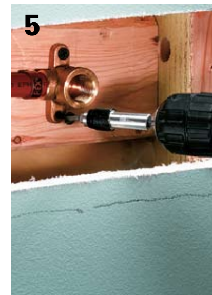
5 At the cooktop, install the faucet union as specified by the manufacturer. Add blocking as needed. The pot filler installed here attaches to a drop-ear L-fitting mounted to the blocking. Apply pipe joint compound to the faucet inlet and thread it onto the L-fitting.
