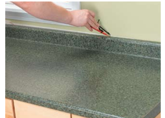
Post-form countertops have a laminate surface that is applied at the factory.
