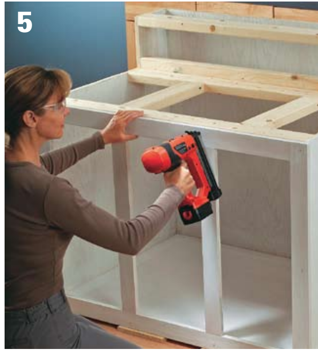
5 Build a face frame from 1 × 2 hardwood to fit the cabinet front. Attach it to the cabinet with 6d finish nails and hang the cabinet doors (we installed three 13"-wide overlay doors).
