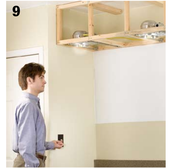
9 Finish installing lights, and then check to make sure they work. Once you've determined that the lights work properly, have the work inspected by an electrician and/or a local building inspector. With approval, you can begin to close up the soffit.
