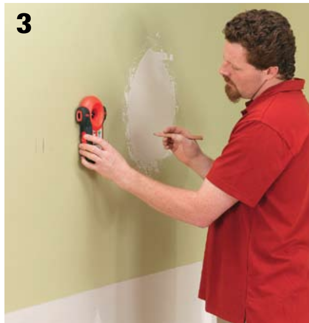
3 Locate and mark wall studs using an electronic stud finder. Cabinets normally will be hung by driving screws into the studs through the back of the cabinets.
