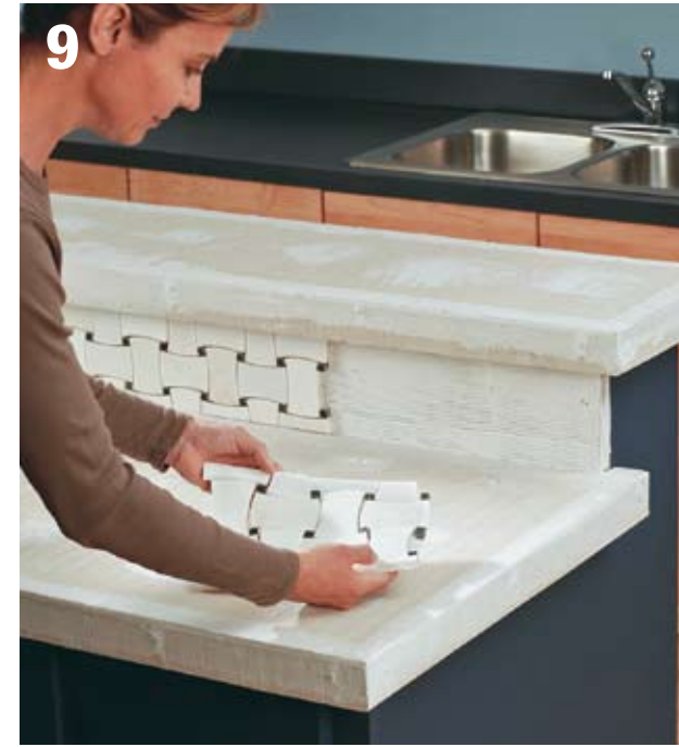
9 Cut mosaic sheets to fit the backsplash area and attach them with thinset adhesive (see Tile Backsplash, page 124).
