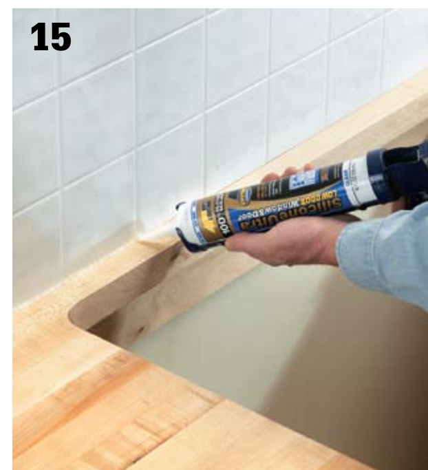
15 Add backsplash of your choice and caulk between the new countertop and the backsplash area with silicone caulk.
