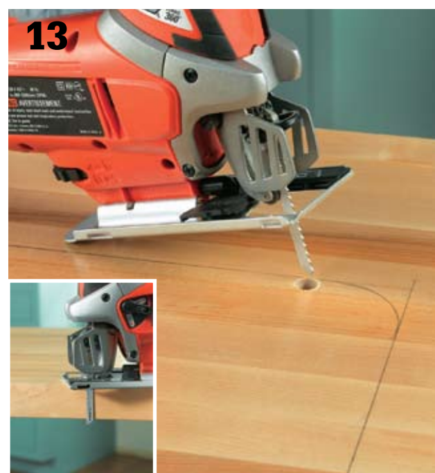
13 If installing a sink in your countertop, start by outlining the sink in the correct position as recommended in the installation material from the sink manufacturer. Mount a downstroke blade into the jigsaw (inset), and drill a starter hole just inside the sink outline. Make the cutout, taking care to stay just inside the cutting line. If you are installing an undermount sink, smooth the cuts up to the line with a power sander.
