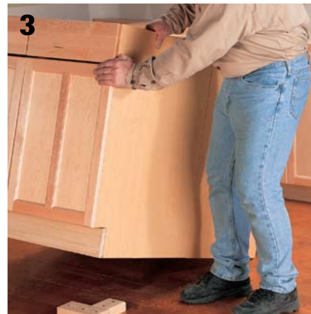
3 Join the two base cabinets together by driving 1 1/4" wallboard screws through the nailing strips on the backs of the cabinets from each direction. Make sure the cabinet sides are flush and aligned. Lower the base cabinets over the cleats. Check the cabinets for level, and shim underneath the edges of the base if necessary.
