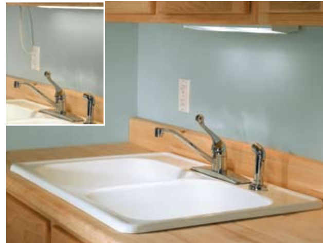
Fluorescent under-cabinet lights run cool (unlike incandescents) and provide the most light with the least amount of electricity. The simplest way to add under-cabinet lighting is with plug-in fixtures (inset), while hard-wired installations don't use up outlet space.
