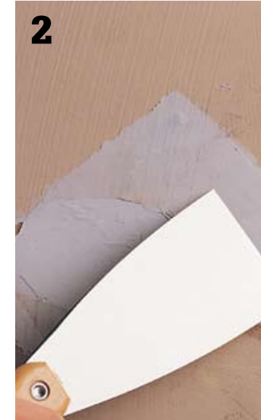
2 Apply spackle to the edges of the chipped paint with a putty knife or a flexible wallboard knife.
