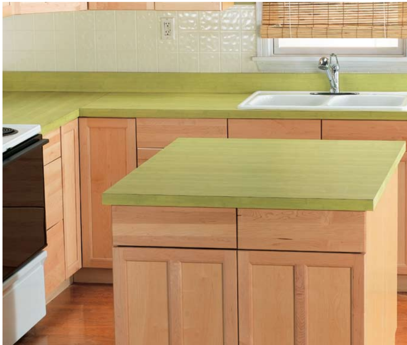
Two base cabinets arranged back-to-back make a sturdy kitchen island base that's easy to install. When made with the same style cabinets and countertops as the rest of the kitchen, the island is a perfect match.
