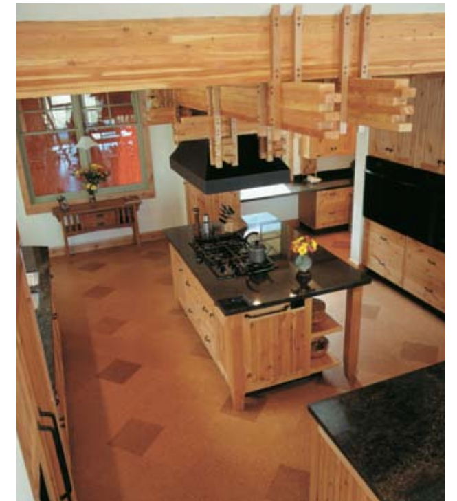
Cork lends a rich, natural character to kitchen floors and helps to keep noise levels down.
