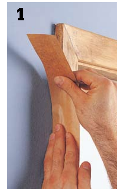
1 Use pregummed paper or wide masking tape to protect wood moldings from paint splatters. Leave the outside edge of the masking tape loose.
