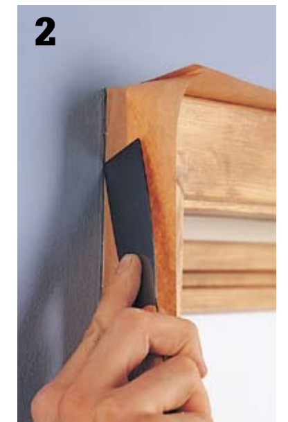
2 After applying the tape, run the tip of a putty knife along the inside edge of the tape to seal it against seeping paint. After painting, remove the tape as soon as the paint is too dry to run.
