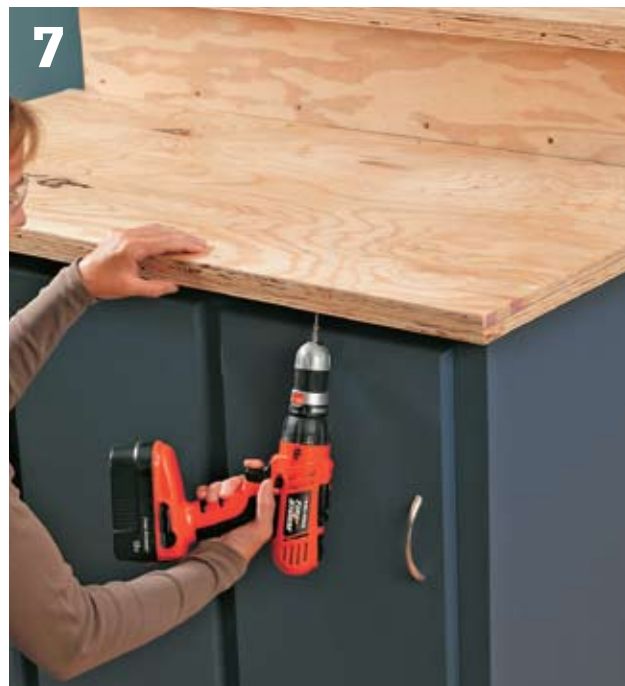
7 Cut 2" wide strips of plywood for buildup strips and attach to the undersides of the subbases with glue and screws.
