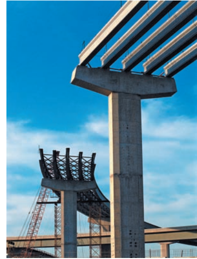
Photo 9.1 A different function M(x) is required in each portion of the beams when a vehicle crosses the bridge.
