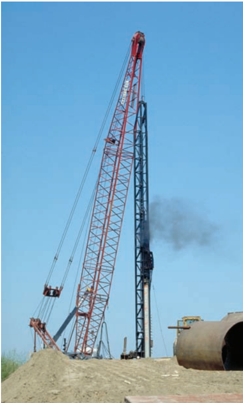
Photo 11.2 Steam alternately lifts a weight inside the pile driver and then propels it downward. This delivers a large impact load to the pile that is being driven into the ground.
