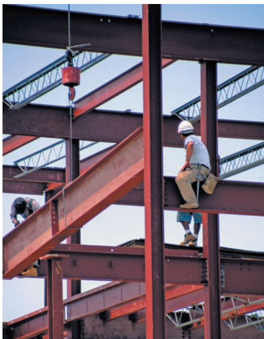
Photo 4.3 Wide-flange steel beams are used in the frame of this building.
