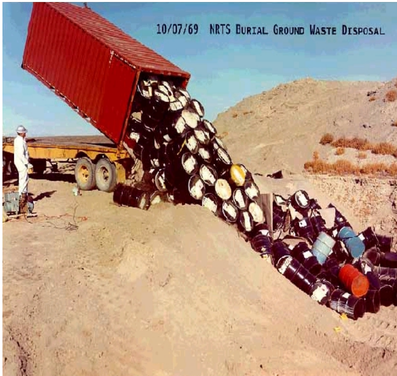
FIGURE 2.1 Before 1970, transuranic and mixed wastes were buried in near-surface trenches. The waste was considered to be permanently disposed, and inventory data are lacking. Source: http://web.ead.anl.gov/techcon/images/ineel3.jpg .
