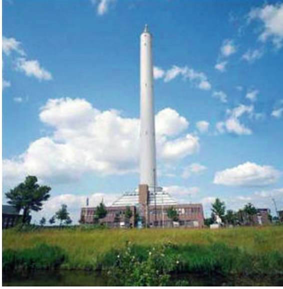
Fig. 13 The ZARM Drop Tower in Bremen, Germany. The 146 m high building protects the free fall facility from atmospheric perturbation and wind. Microgravity levels of 10^{-5} g are obtained during 4.7 s in drop mode and 9.5 s in catapult mode. (Photo: ZARM)
