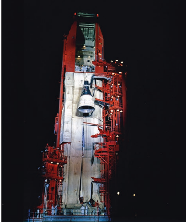
Gemini 3 is hoisted to the White Room on Pad 19. (Courtesy Ed Hengeveld)
