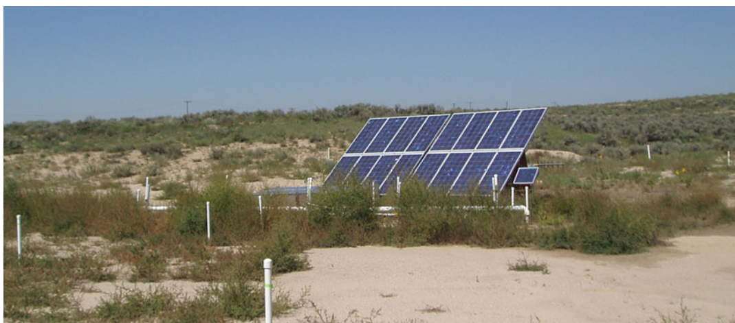
Figure 17.4. Solar photovoltaic powered e-barrier for treatment of energetic compounds at the Pueblo Chemical Depot.
