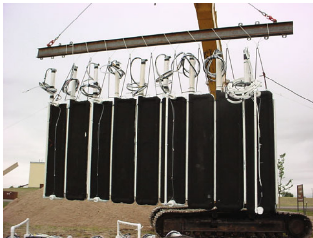
Figure 17.10. Nine e-barrier modules prior to installation (from Sale et al., 2005).
