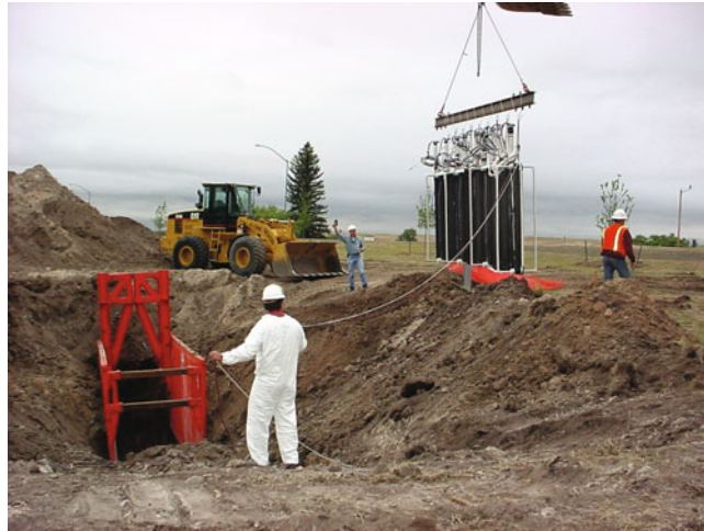
Figure 17.8. Installation of the e-barrier at F.E. Warren AFB.
