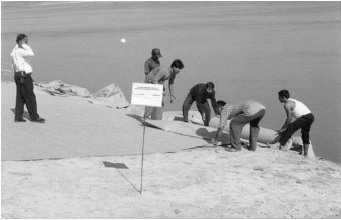
Fig. 12 Laying of jute nonwoven fabric rolls on the river bank
