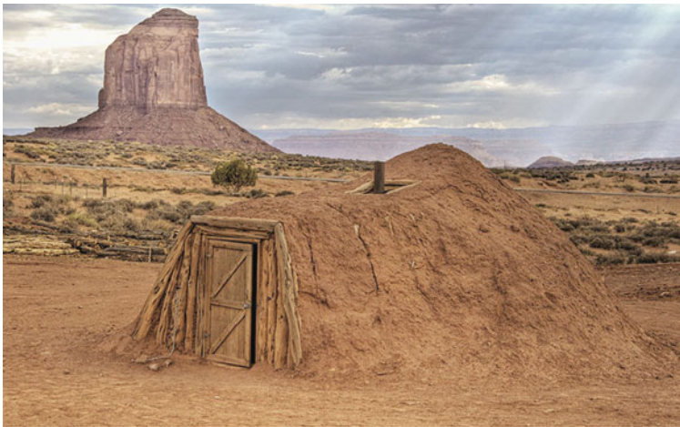
Fig. 7.8 The Navajo hogan, used by present-day Navajo, embodies the principles of the Navajo cosmology in its design and is aligned so the entrance faces east ( image source : photo by Wolfgang Staudt from Saarbruecken, Germany, at http://commons.wikimedia.org/wiki/Image:Navajo_Hogan,_Monument_Valley.jpg )
