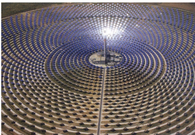
Fig. 7.6 Gemasolar plant of Torresol Energy in Andalusia, Spain (Torresol Energy) (see endnote 51)
